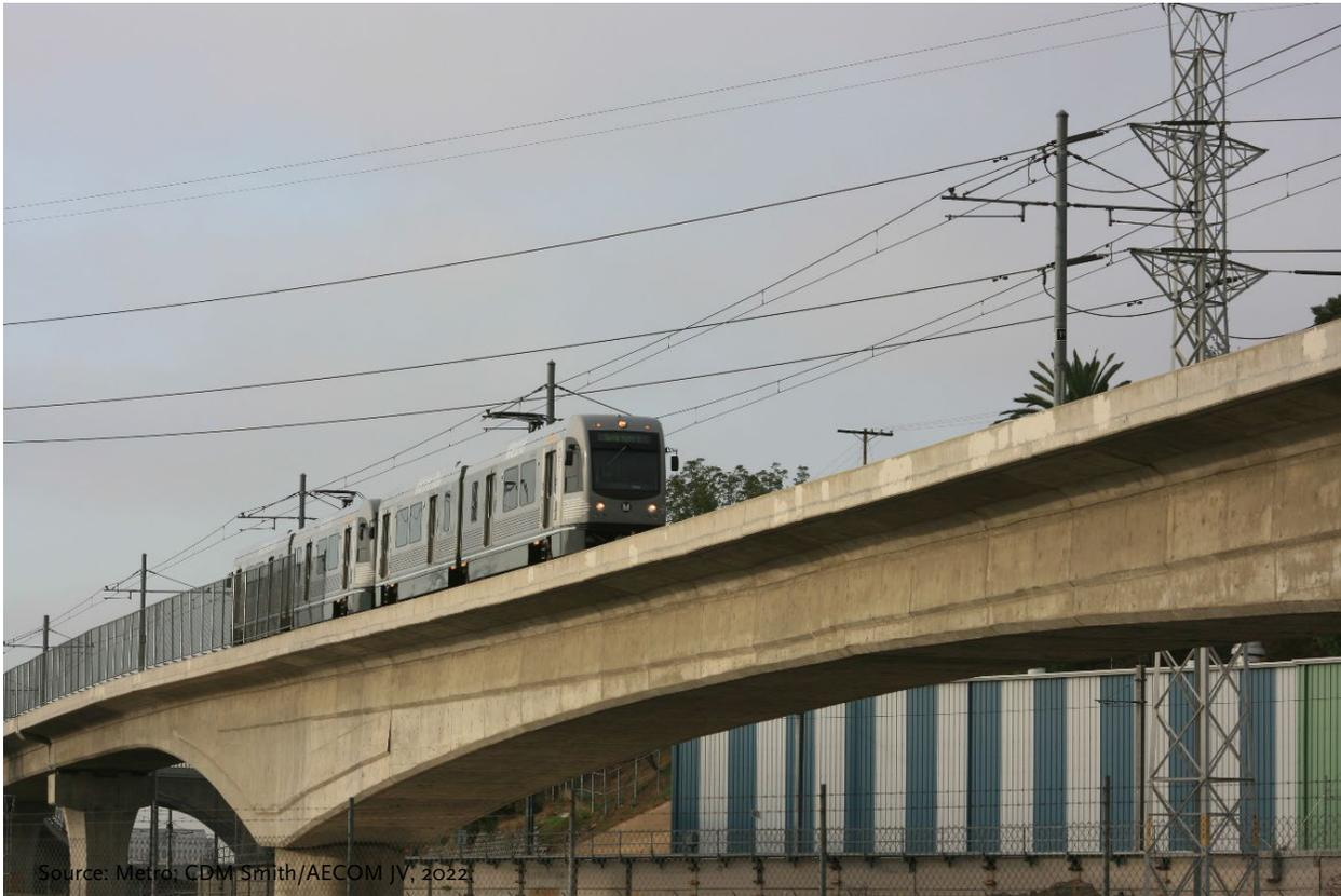
**Figure 3.5. Example of an Aerial Structure**
