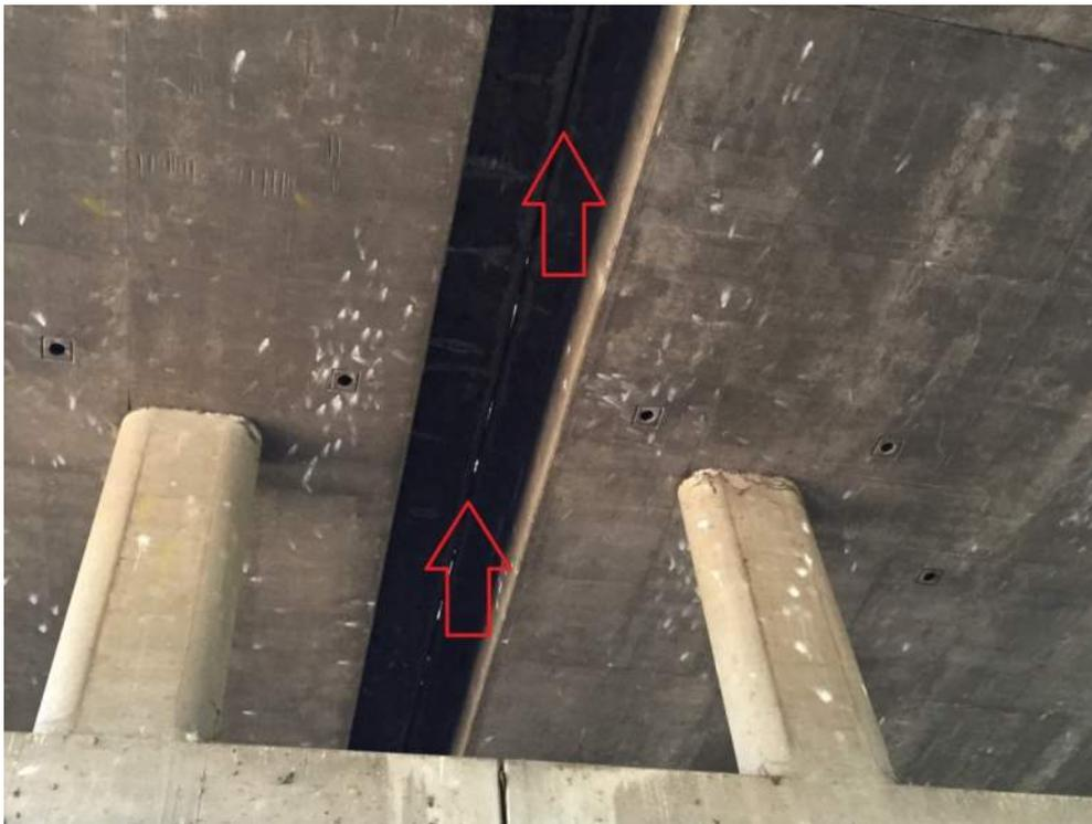
Photo 12: Underside of the SR-60 Bridge with expansion joint running down the center of the bridge with sealed areas and unsealed areas; view facing west
