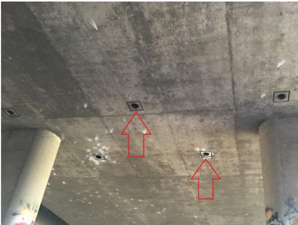
Photo 14: Vent holes on the underside of the SR-60 Bridge providing access to the bridge interior; view facing west
