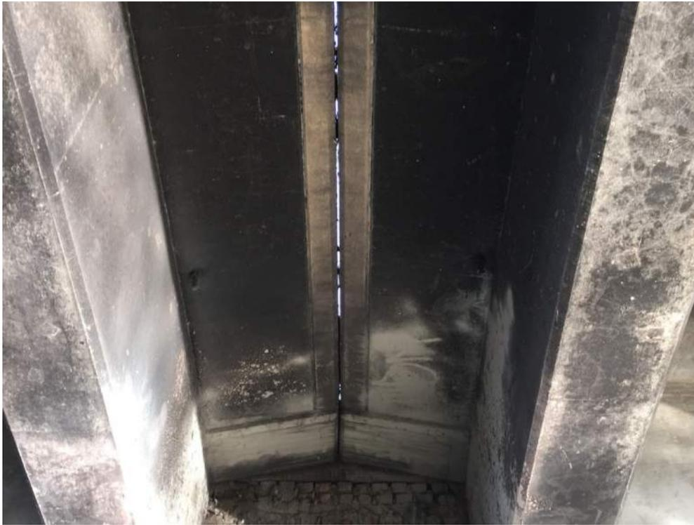
Photo 7: Washington Boulevard Bridge over the San Gabriel River with expansion joint down the center of the bridge open to roadway surface (not suitable for bat roosting); view facing east
