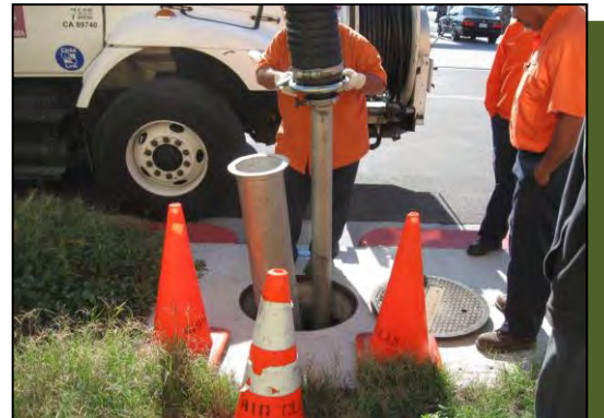
Insertion of vacuum hose into separation chamber.
