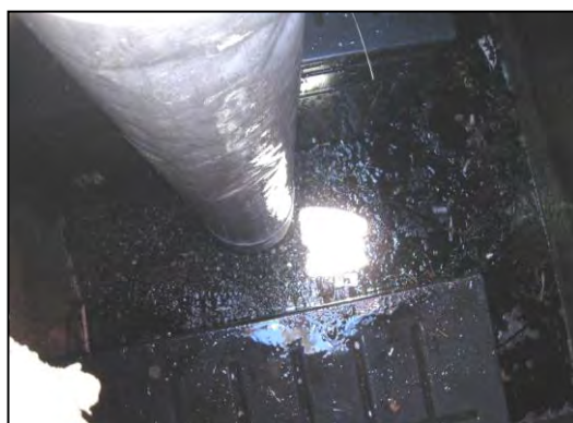
Removal of trash, sediment and debris.
