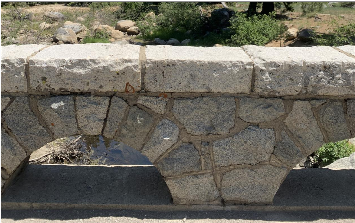
Source: Photograph taken by Ascent Environmental in 2021. Stone Railing of SR 89 Bridge over Meeks Creek
