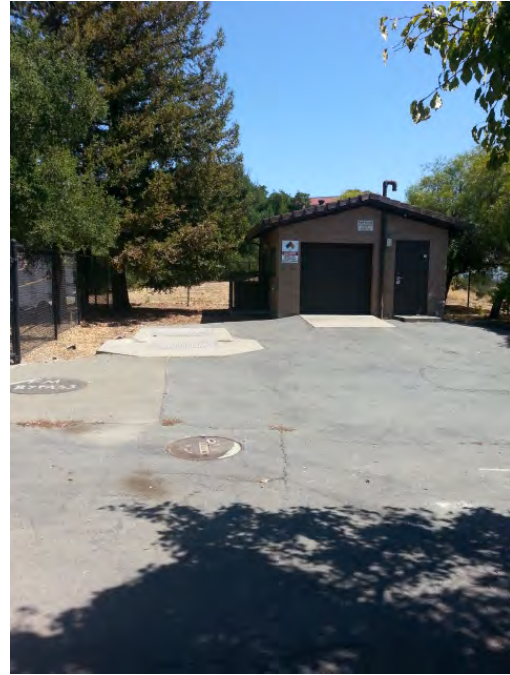
PHOTO 6 – ADJACENT PUMP HOUSE.
