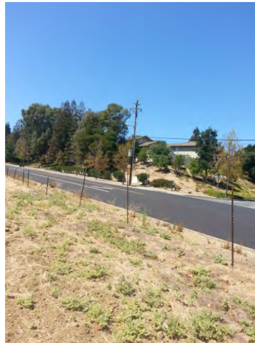
PHOTO 4 – VIEW TO NORTHWEST.
