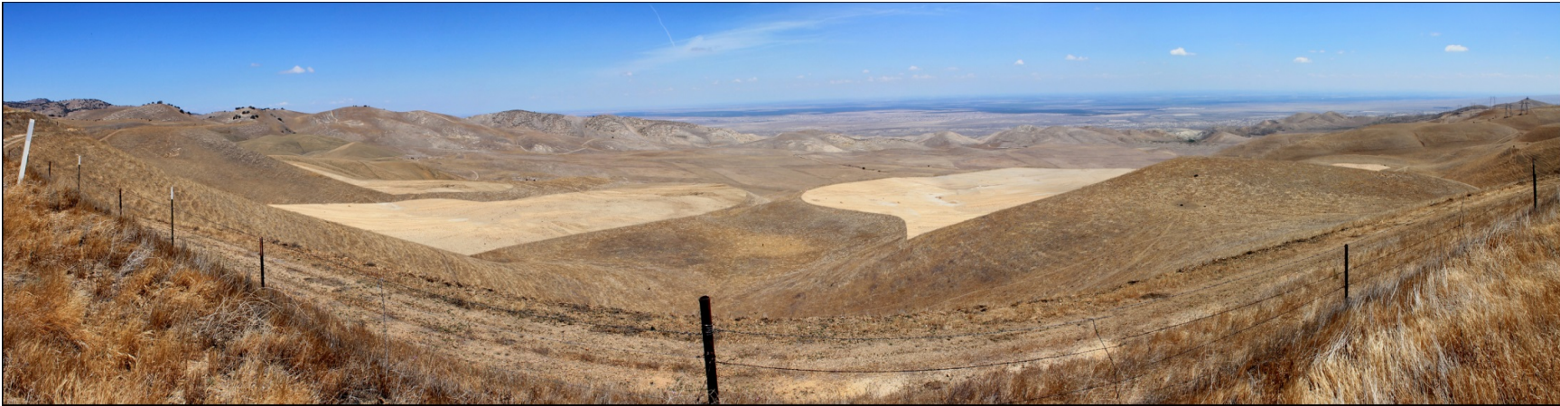
Figure 4.1-11 KVA-2: Mine Areas 1, 2, and 3 Have Been Fully Mined but Reclamation Has Not Commenced
