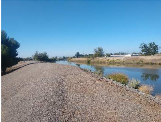
Figure 19 – View of western boundary facing south.
