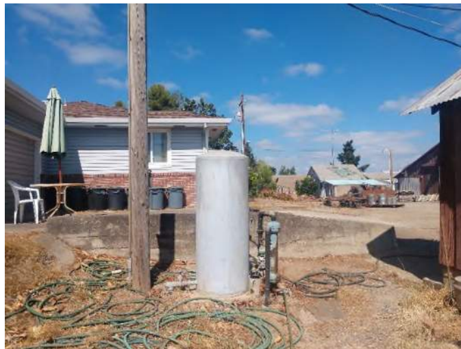
Figure 16 – View of domestic well near residential structure.
