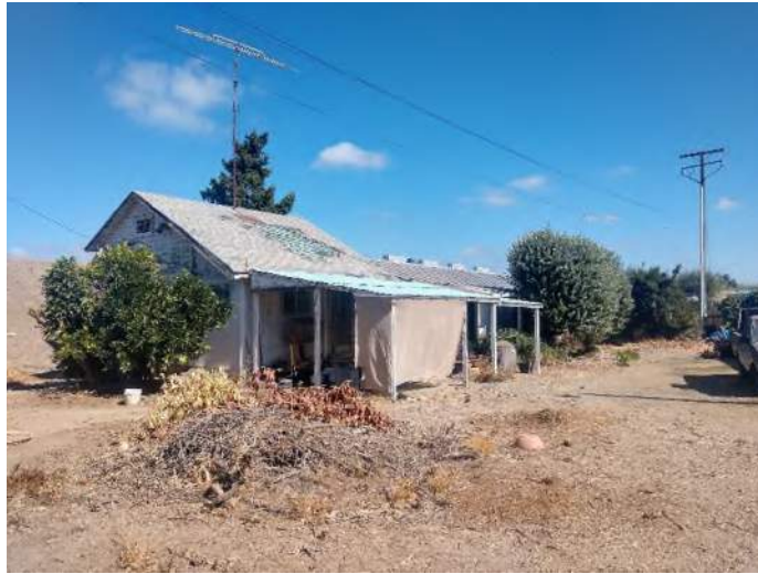
Figure 15 – View of abandoned house structure facing northwest.
