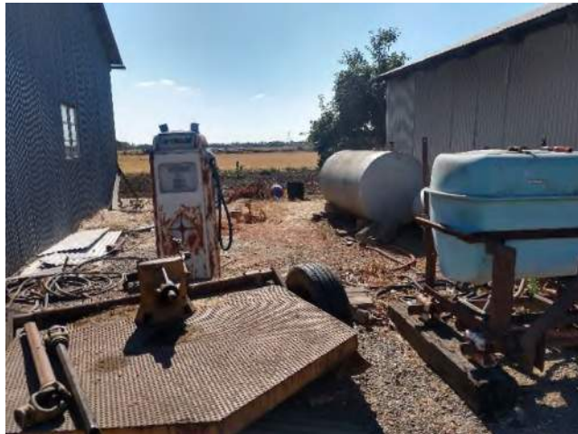
Figure 4 – View of aboveground storage tank with underground piping to gas dispenser.
