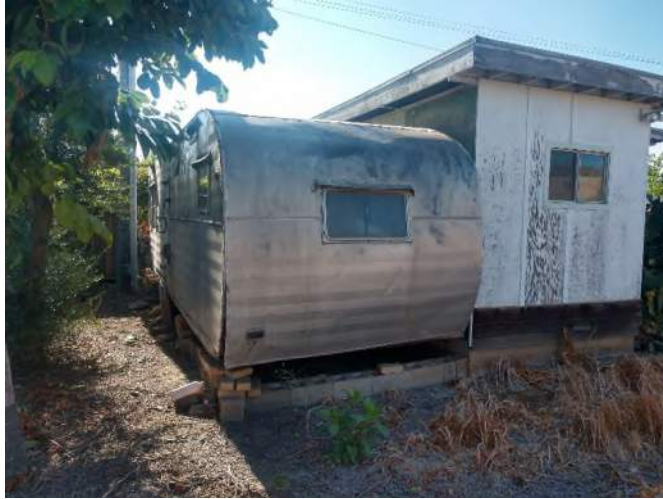
Figure 13 – View of abandoned trailer structures in the northwest corner of site.
