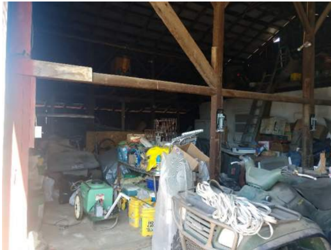
Figure 12 – View of inside of barn.
