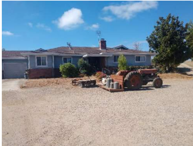
Figure 7 – View of residence, facing south.
