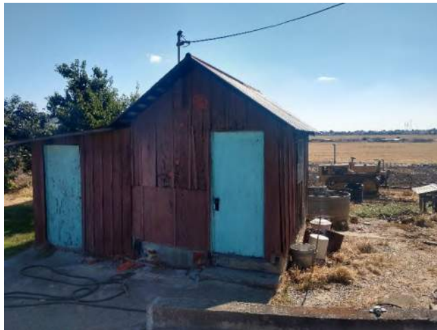
Figure 8 – View old bath house, facing east.
