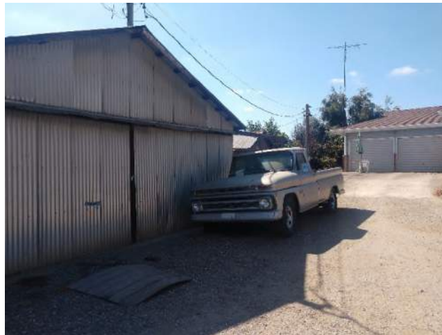
Figure 6 – View of shop looking south, with residential garage in background.
