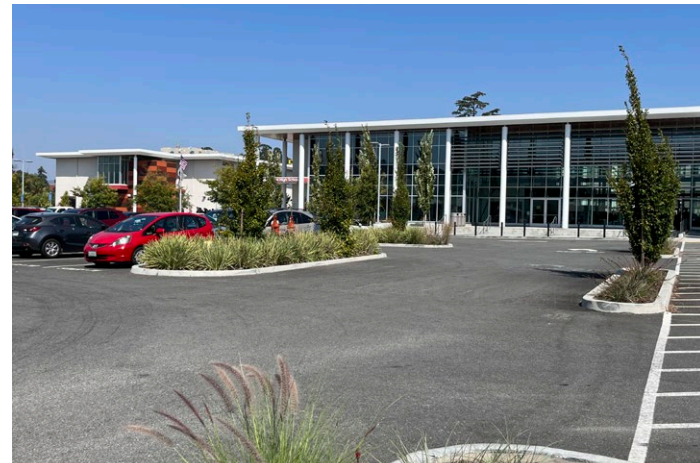
d. View of newly constructed Student Commons as seen from 3rd Street
