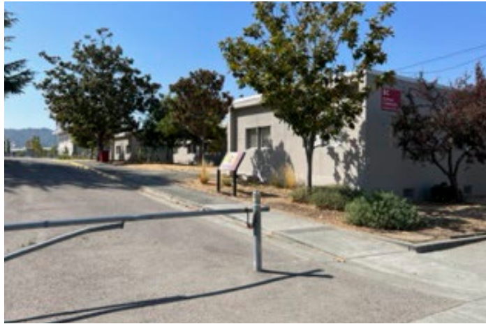
a. View from Mission Avenue to the south looking towards Science Building
