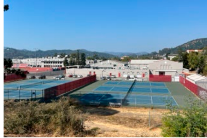
b. View west towards Large Gym and Aquatics Center from Mission Avenue
