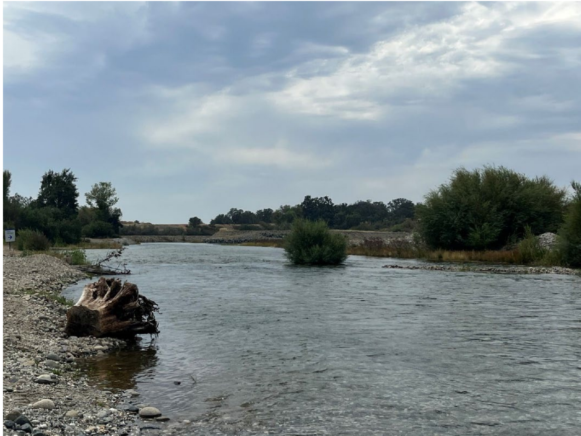
Figure 5. View of the south channel after excavation in 2022. One of the three root wads that was placed in the south channel in 2018 can be seen on the left side of the picture.
