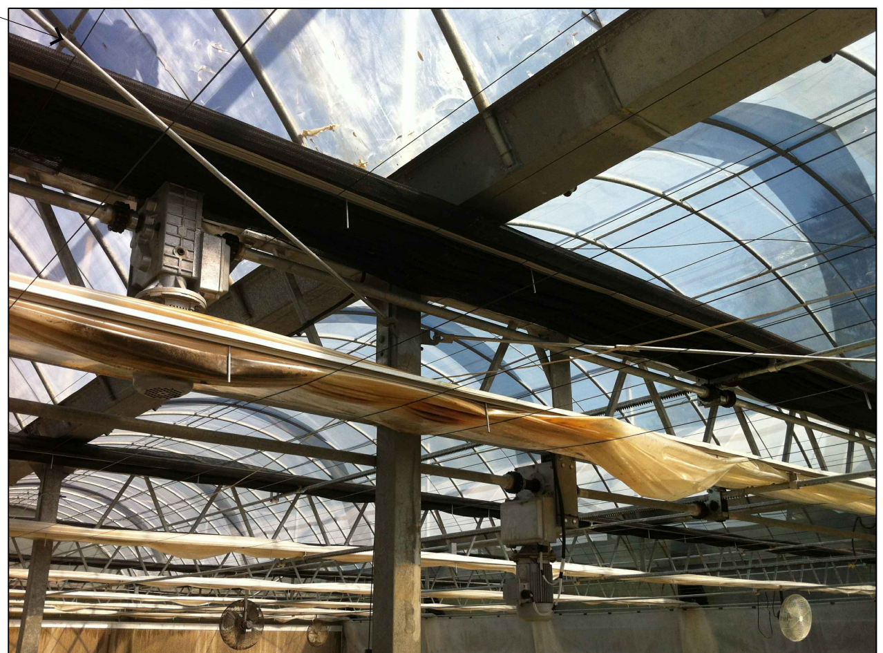
COLLUM / X-BRACE / TRUSS ASSEMBLY
