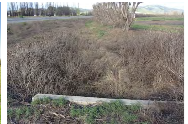
④ Looking west along drainage ditch from culvert under Bolsa Road
