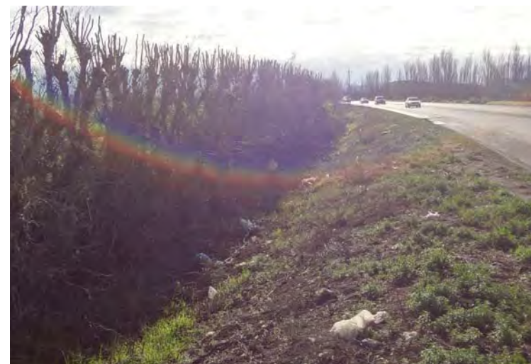
① Drainage ditch on north side of SR-25, looking east
