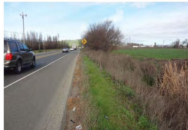
② Drainage ditch and wetland on north side of SR-25, looking west
