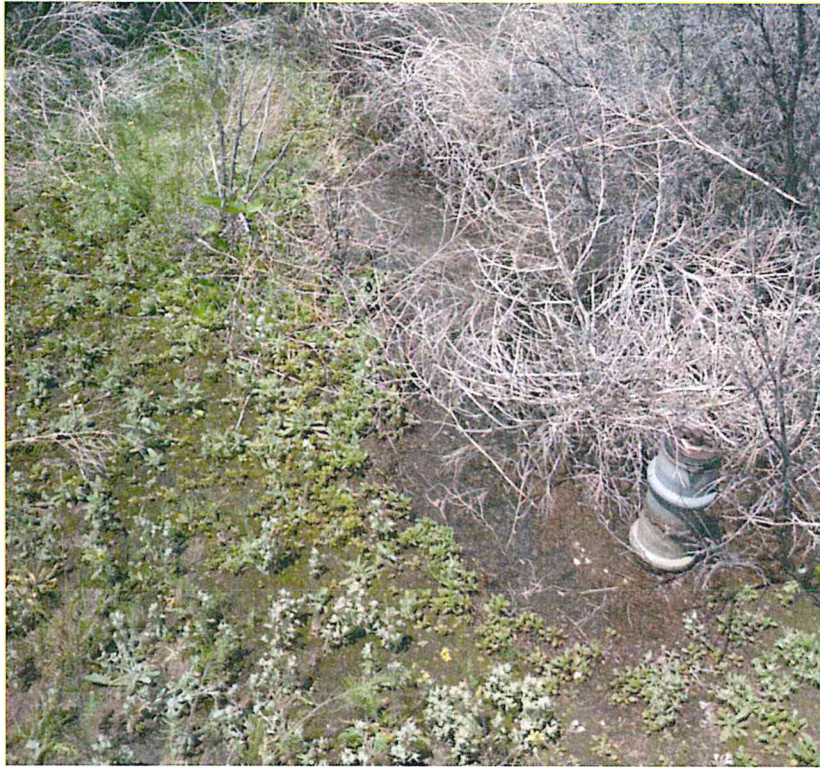
Irrigation valve upslope of culverted driveway crossing, view to northwest
