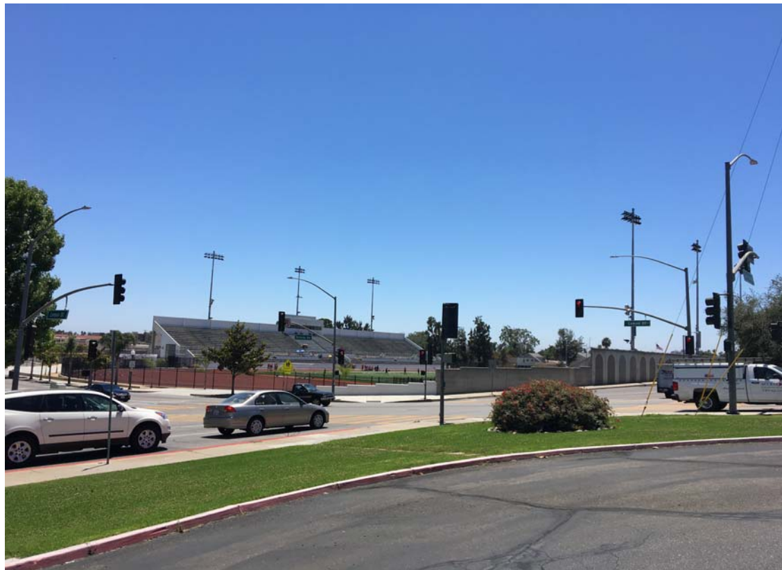
Photo K: View west from North Lemon Street toward Fullerton High School Stadium
