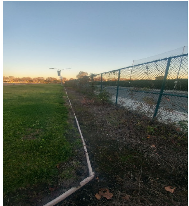
Drainage Area 2 (South of Sherbeck Field)
