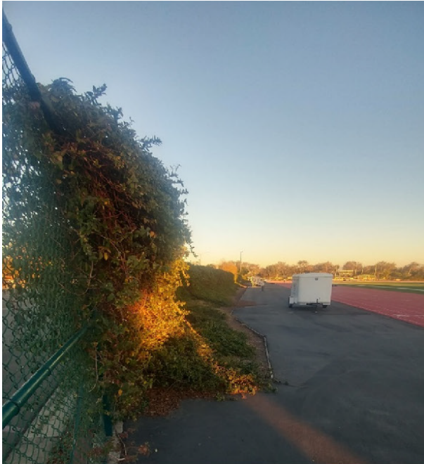
Drainage Area 1 (North of Sherbeck Field)
