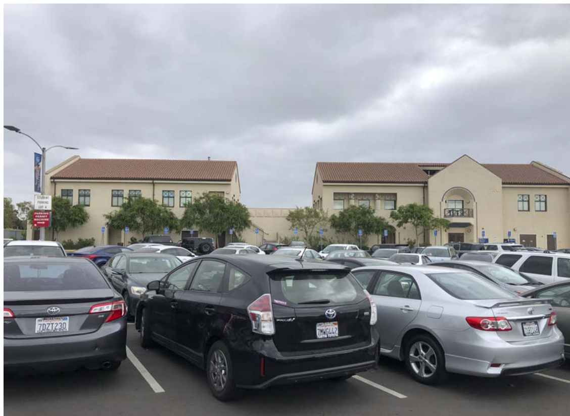
Photo G: View east from Student Parking Lot 4 towards west elevation of field house structure
