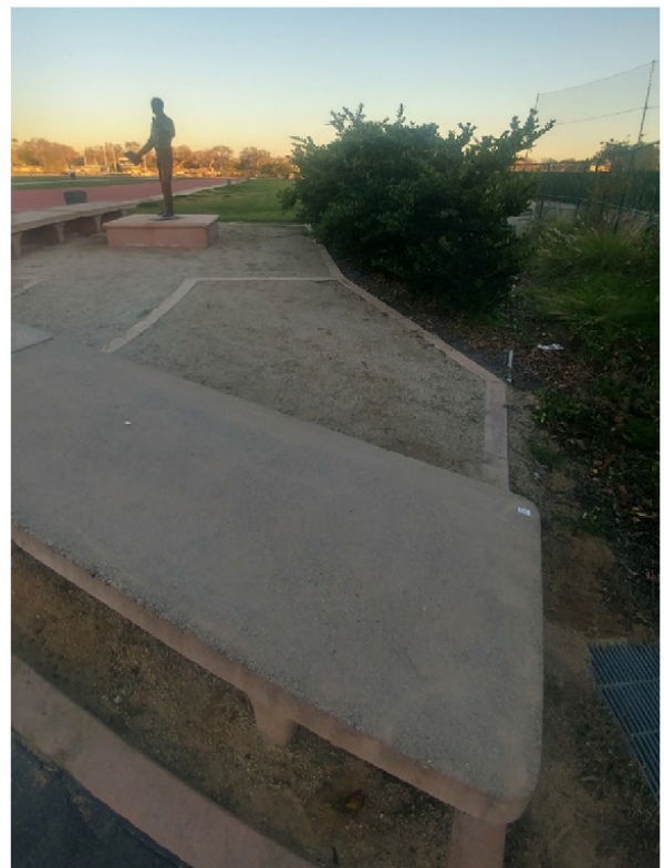
Drainage Area 2 with existing catch basin used for drainage
