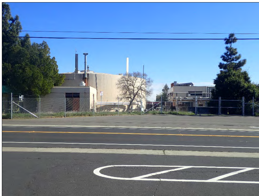
Photograph 2. Wastewater treatment plant processing tanks; eastern elevation facing South River Road. Image taken February 2018; view west.
