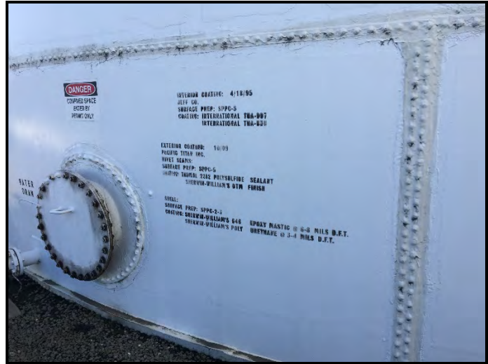
Photographs 6 and 7. Close-up images of riveted tank seams, characteristic of tanks built in 1950 and earlier. Images taken February 2018.
