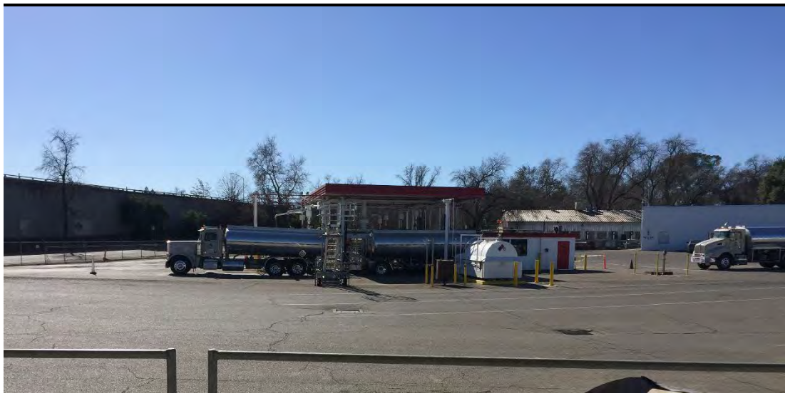
Photograph 5. Phillips 66 parcel showing main truck fueling structure. Front Street and the raised Interstate 5 freeway are at the left of the image. The warehouse at the back of the image sits at the southern boundary of the parcel. Image taken February 2018; view southwest.
