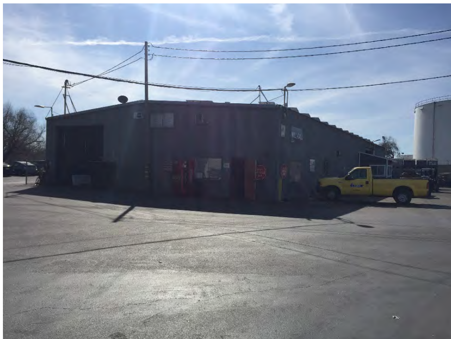
Photograph 5. Main warehouse building on parcel; view south.
