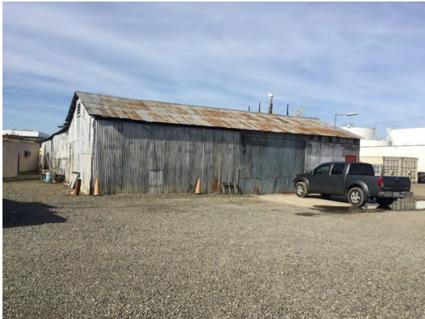
Photograph 2. L-shaped warehouse building on parcel; view northwest.
