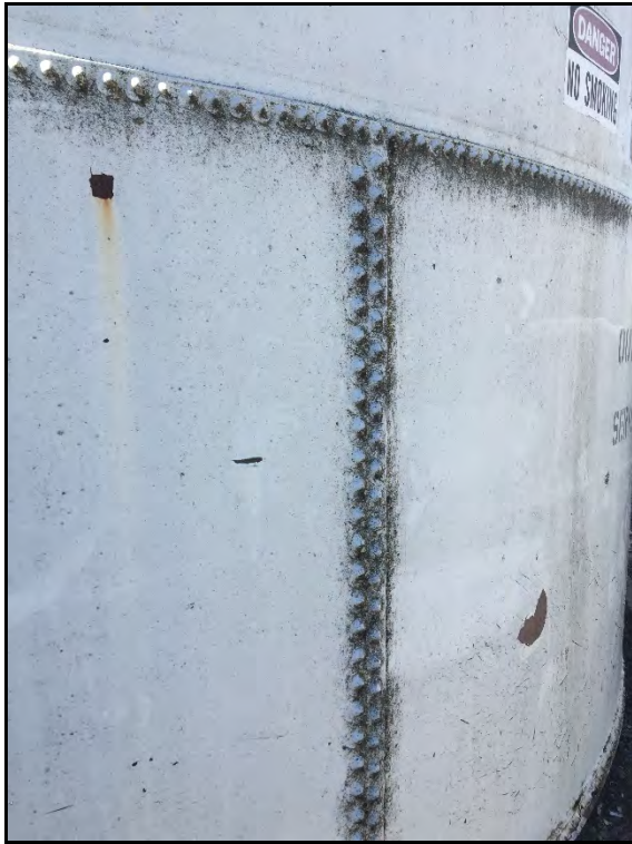
Photographs 6 and 7. Close-up images of riveted tank seams, characteristic of tanks built in 1950 and earlier. Images taken February 2018.
