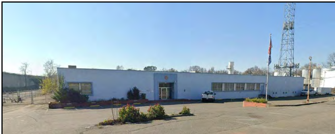
Photograph 3. Phillips 66 offices building dating to 1955; northern elevation showing single-story building with flat roof and multi-pane fenestration. Image February 2020; view southwest.
