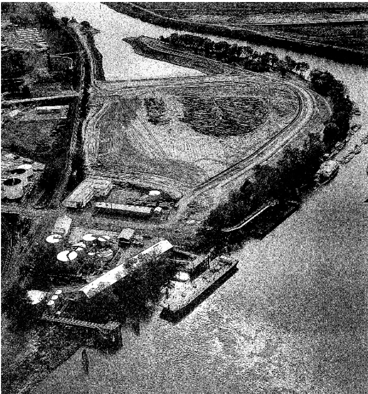
Exhibit 3. Historical photograph (1957) of the Tidewater Company's operations at the Broadway wharf and grading of the land that would become Miller Park.
