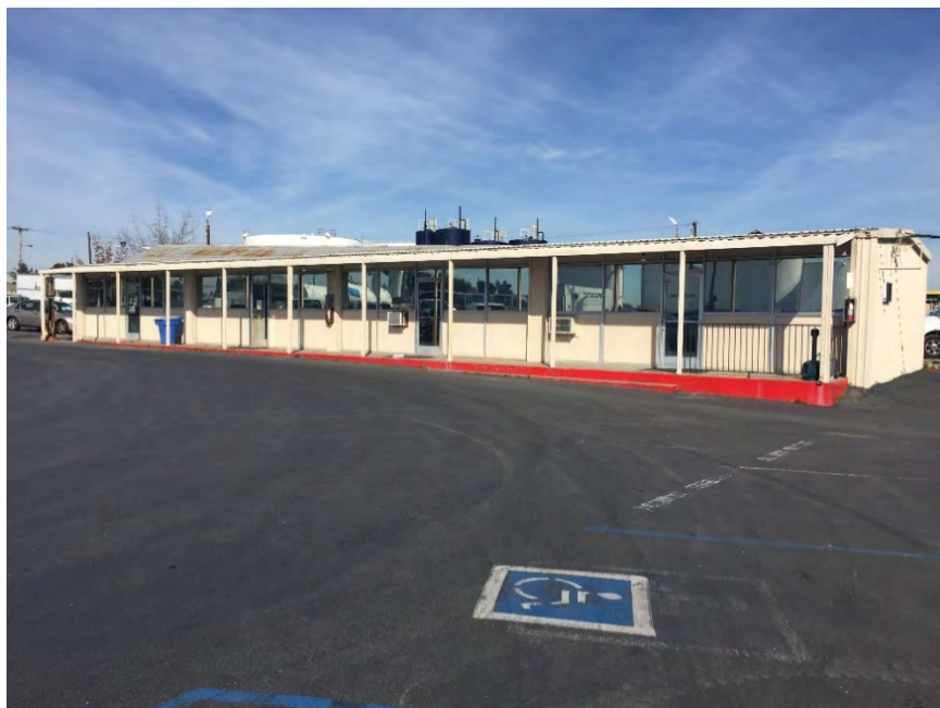
Photograph 3. Office building on parcel; view northwest.
