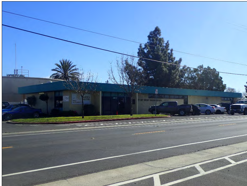
Photograph 1. Wastewater treatment plant services building; eastern elevation facing South River Road. Image taken February 2018; view west.
