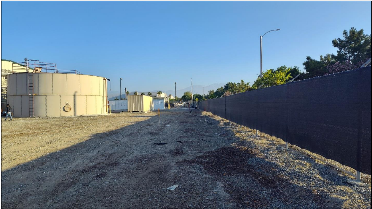
Figure 4. Typical landscape at the proposed lift station site on Mountain Avenue, view to the north. (Photograph taken on September 8, 2023)
