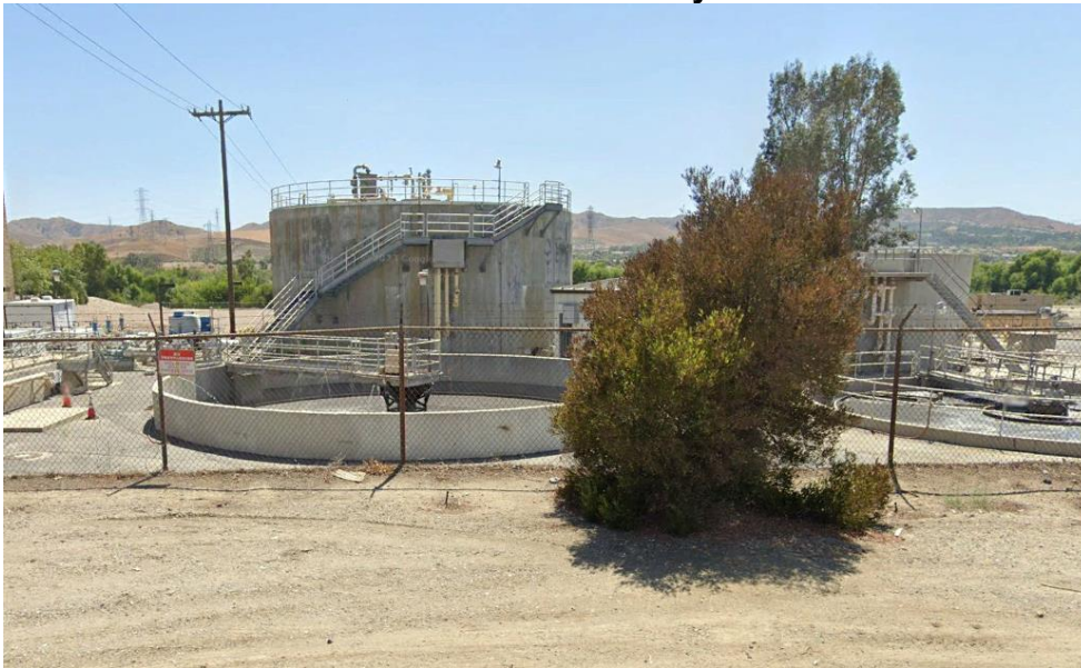
View of RP#2 Facility
