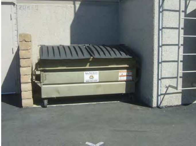
5) View of typical trash enclosure.
