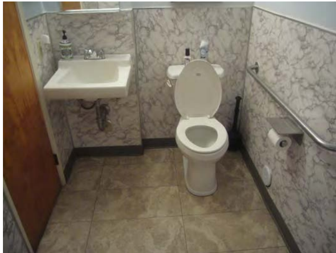
7) View of a typical restroom.
