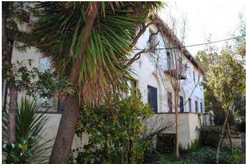
Partial view of Building 1, looking southeast (current)
