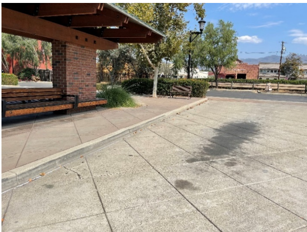
Visible staining was only observed at the center drive aisle of the San Dimas Park & Ride.
