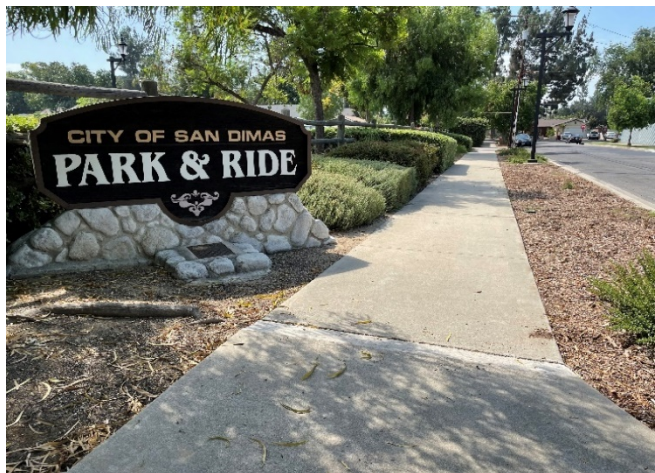
Sidewalks along the border of the Subject Property demonstrate negligible cracking.
