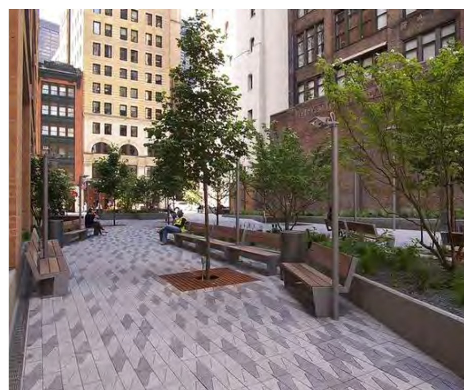
OUTDOOR UNIT PAVING ON PEDESTAL SYSTEMS
