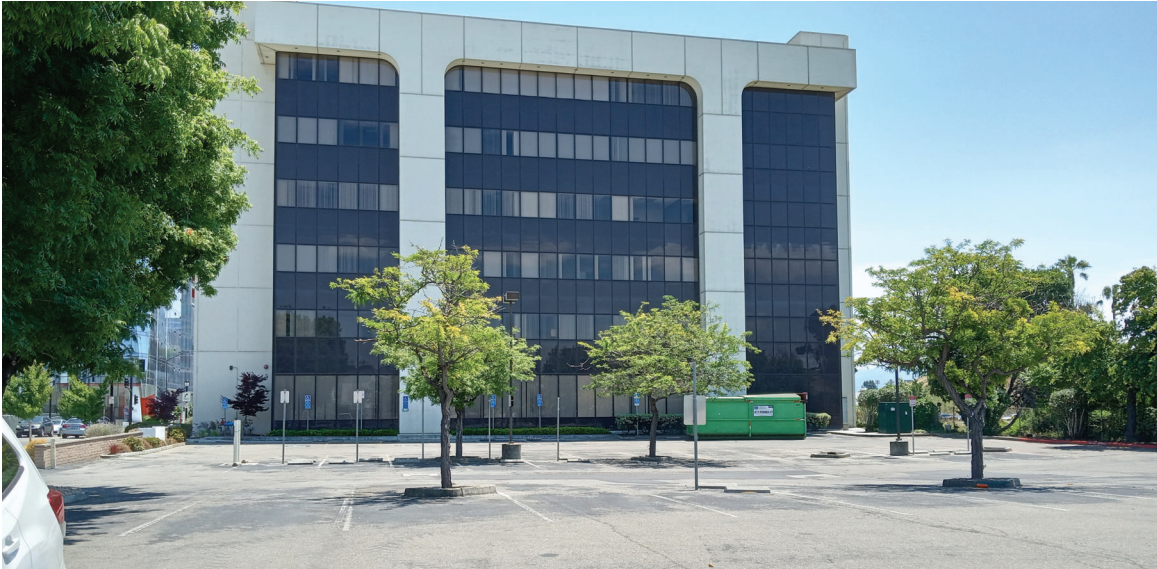
Photo 7: View of parking lot South of Project Site looking South
