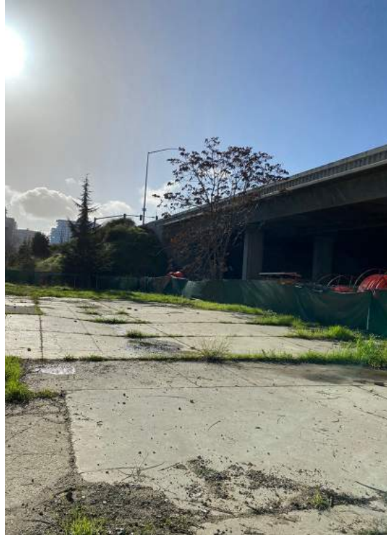
FROM BASSETT ST. LOOKING TOWARD 87 GUADALUPE PARKWAY - SHOWING OFFSITE INVASIVE AILANTHUS ALTISSIMA
