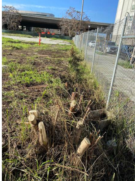
FROM CORNER OF TERRAINE ST. AND BASSETT ST. LOOKING DOWN BASSETT - SHOWING STUMPS OF REMOVED SHRUBS
