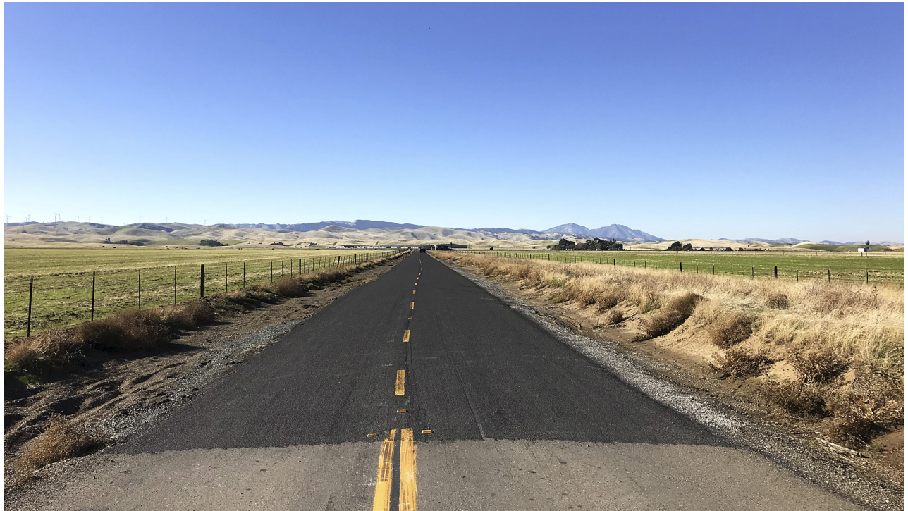
Key Observation Point 3 - Existing Conditions
