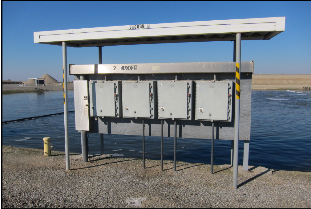
Figure 5-10. Electrical – Typical Lagoon Switch rack
