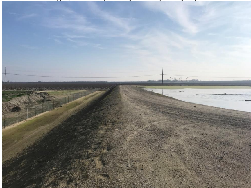
Photograph 4: Reference photo WWTP central north on site, facing east. GPS Coordinates: 35.684614, 119.278074. Photograph taken by M. Wayman on January 17, 2022.
