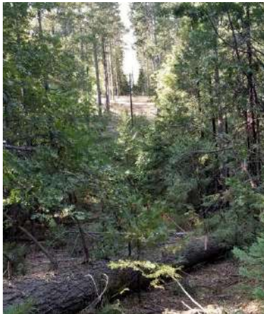
Figure 6: Image of Veg Related Damage in Shasta County – Fallen Tree That Caused Two Primary Overhead Wires Down
