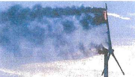
Fire safety in wind turbines – there is more to kn... Engineering and Technology
