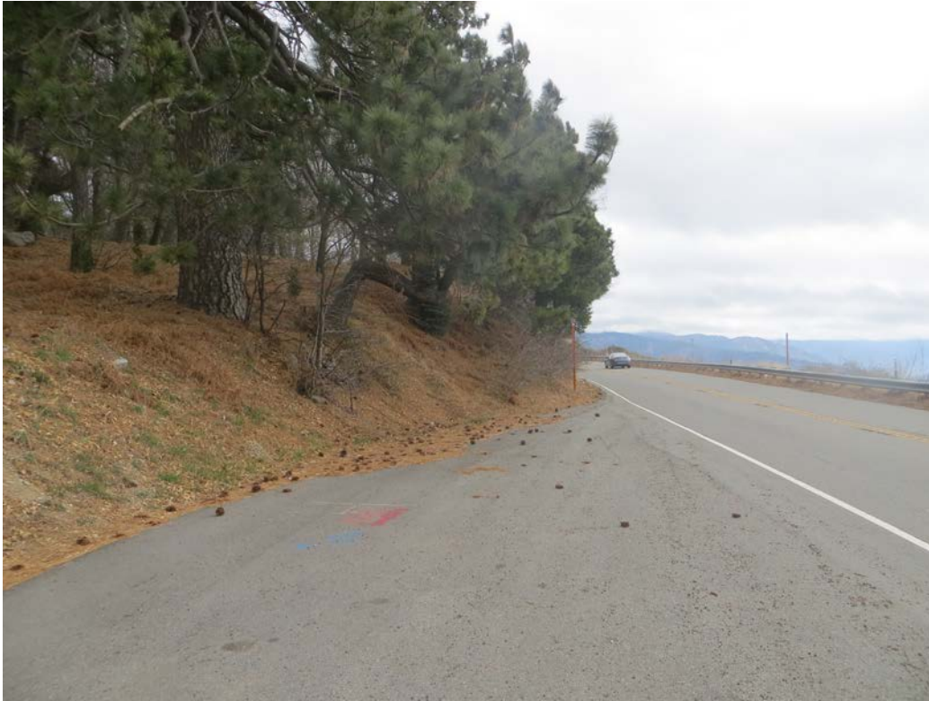
Photograph 9: Looking east at State Route 18 which abuts the southern boundary of the project site.
