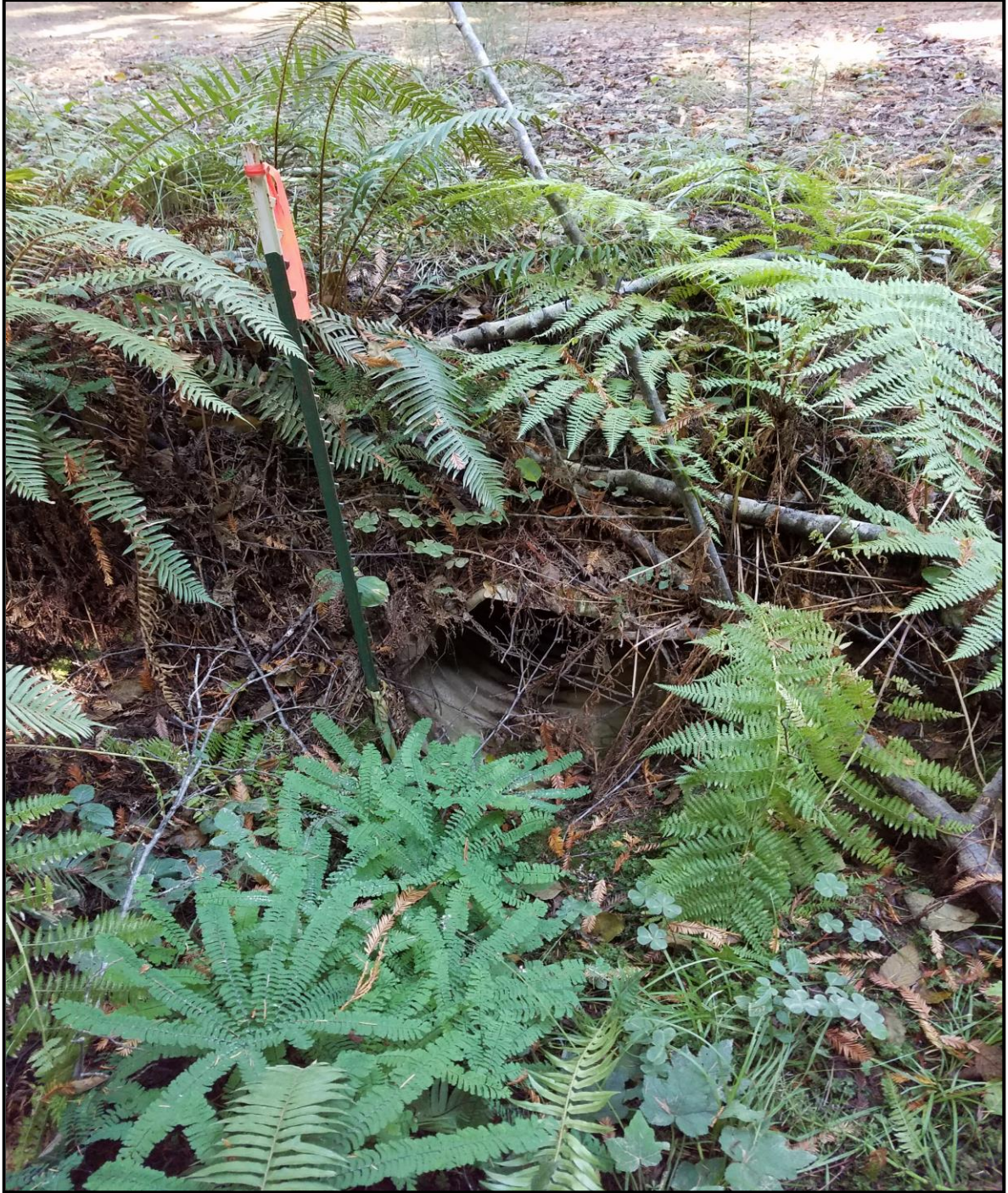
Figure 6. Road 720 Watercourse Crossing (Culvert Replacement and Upgrade)
