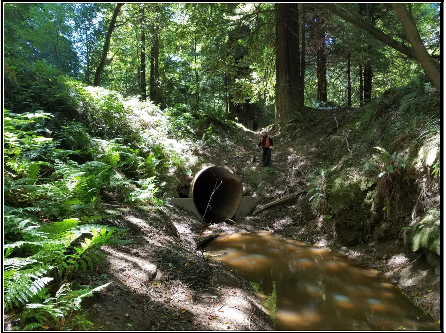
Figure 4. Road 720 Railroad Gulch Crossing (Replacement and Upgrade).
