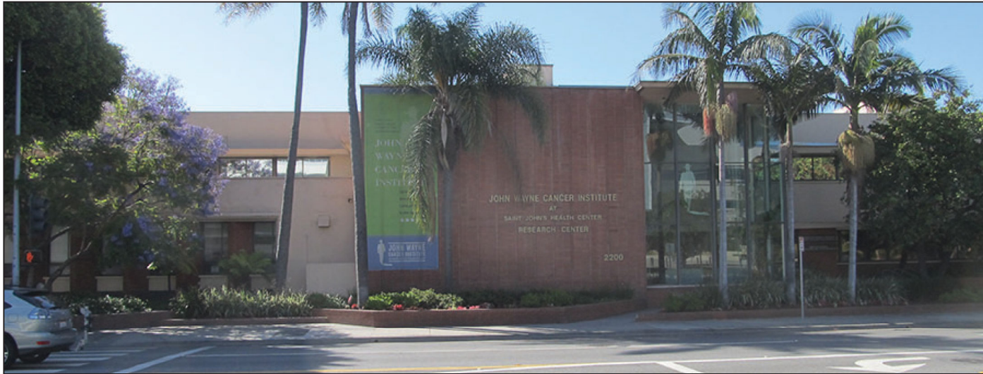
PHOTOGRAPH 5: View of the John Wayne Cancer Institute on Site S4 from Santa Monica Boulevard looking south.
