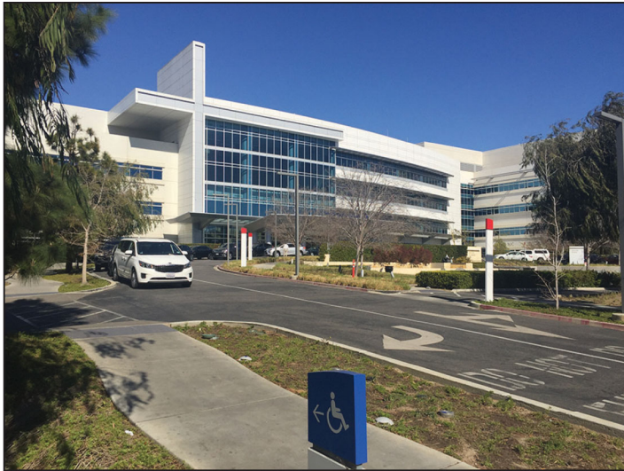
PHOTOGRAPH 1: View of the semi-circular driveway, Mullin Plaza and the west wing of the PSJHC.
