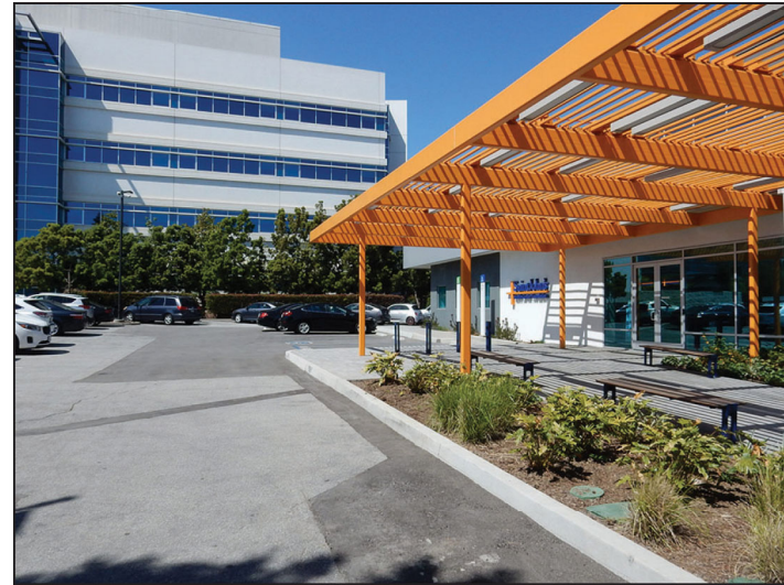
PHOTOGRAPH 2: View of the parking lot and office building on Site 2D/E from Santa Monica Boulevard.
