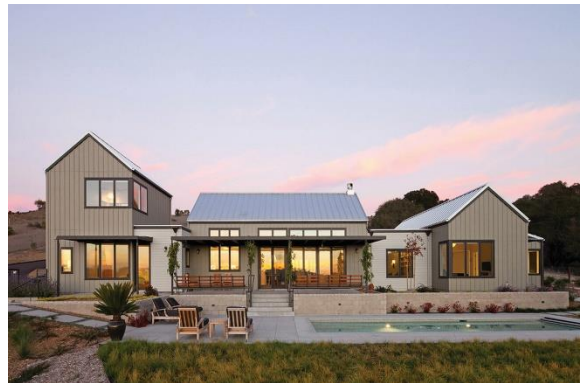
Figure 12 – Typical Farmhouse Character
