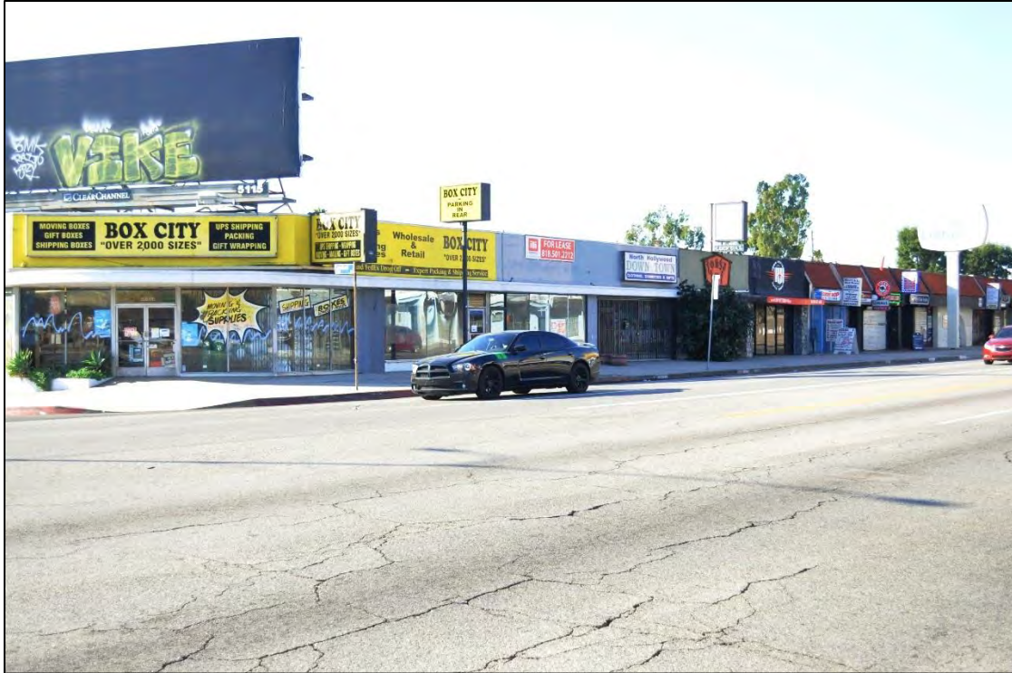
South West Corner of Victory Blvd and Coldwater Canyon Ave – Commercial Building (Strip Mall) – DSC0061
