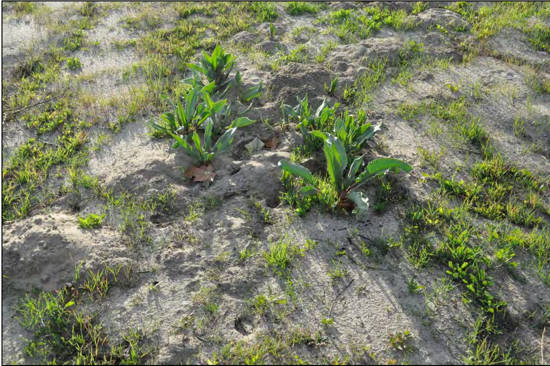
Vegetation within Whitnall Highway Utility Corridor South of Victory Blvd – DSC0030
