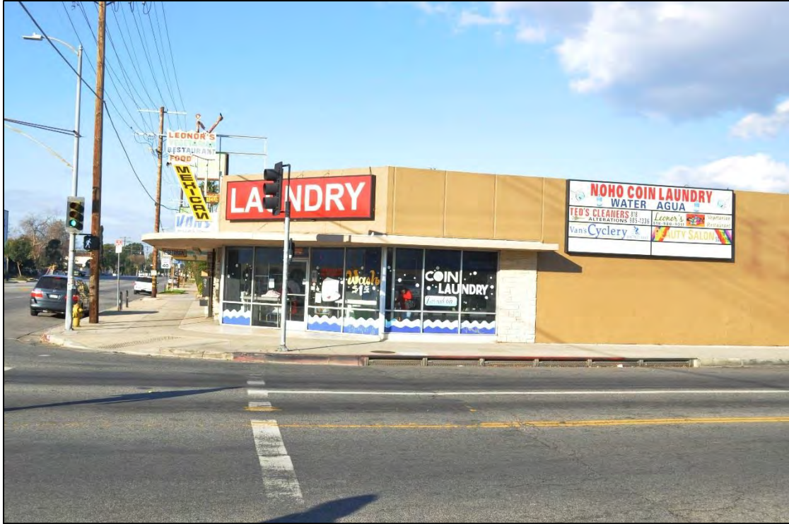
11401 Victory Blvd-North West Corner of Tujunga Ave and Victory Blvd – Commercial Building (Strip Mall) – DSC0044
