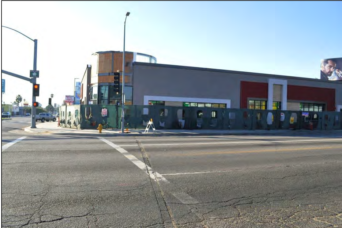
South West Corner of Victory Blvd and Lankershim Blvd – Commercial Building – DSC0053
