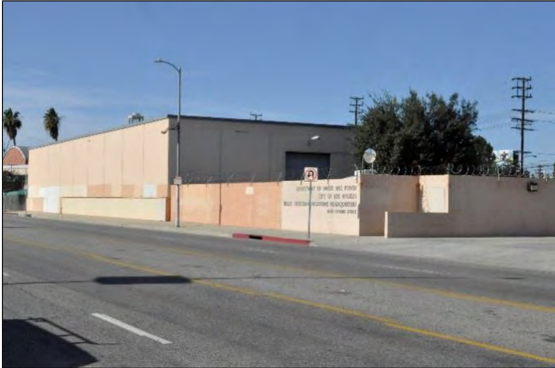
14453 Oxnard St. – Utilities Building - DSC0113
