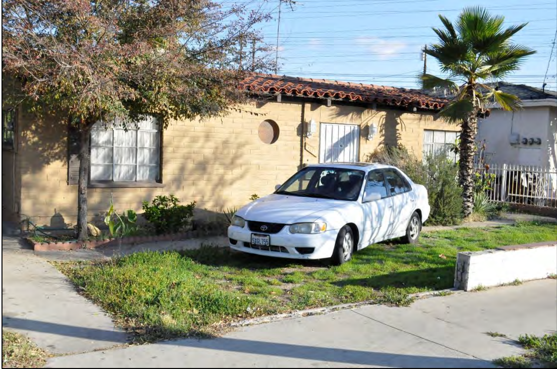
11241 Victory Blvd – Single-family home - DSC0038
