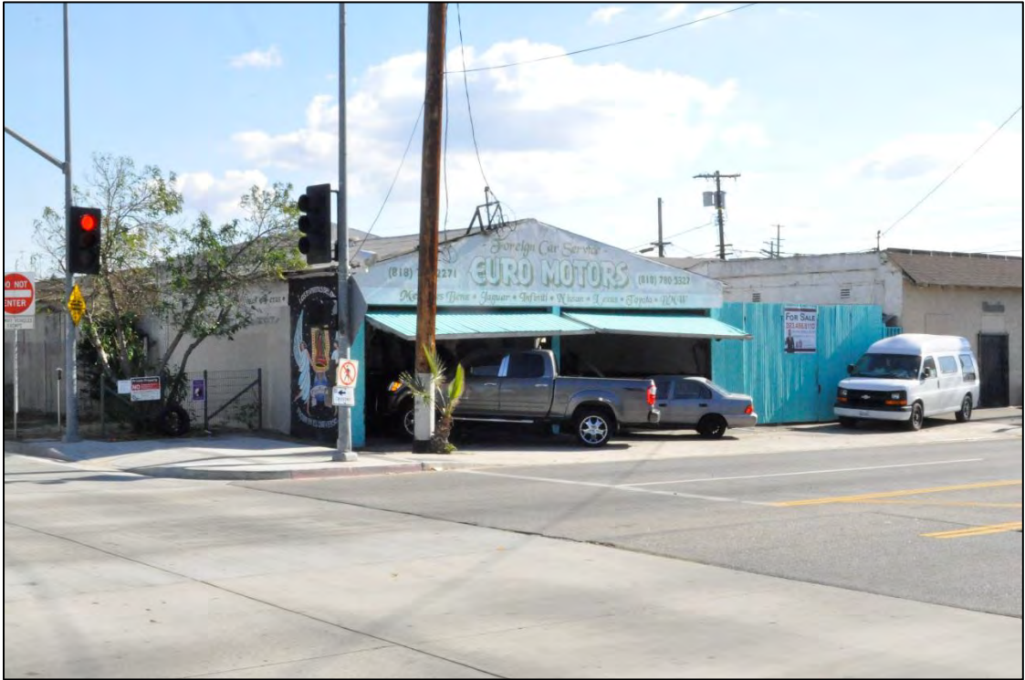
6030 Kester Ave – Commercial Building – DSC0107
