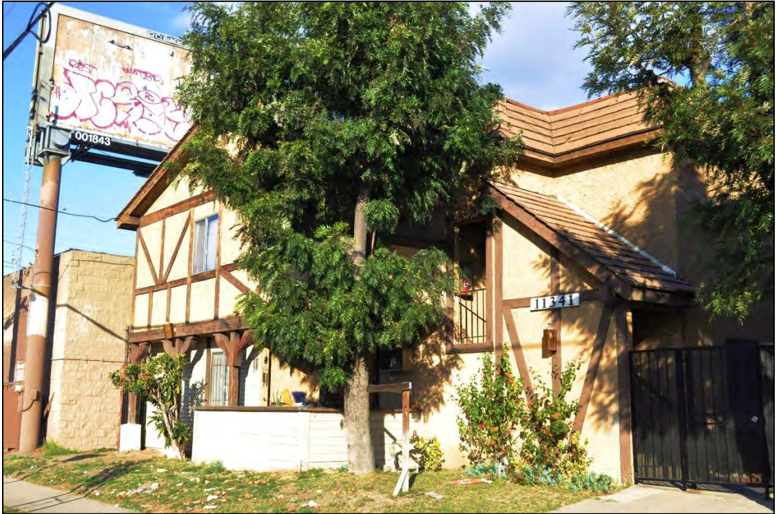
11341 Victory Blvd – Apartment Building -DSC0041
