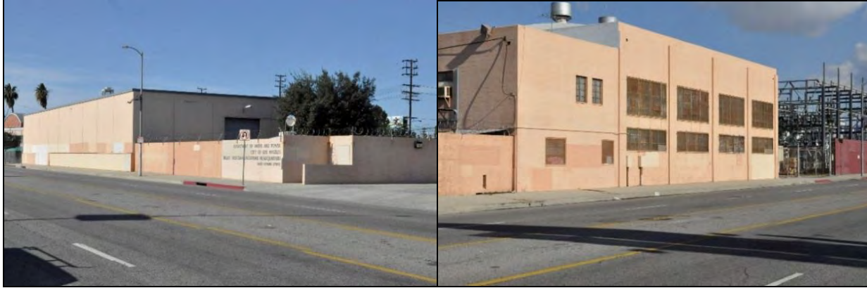
Figure 19. Valley Communications Headquarters operated by the Department of Water and Power
