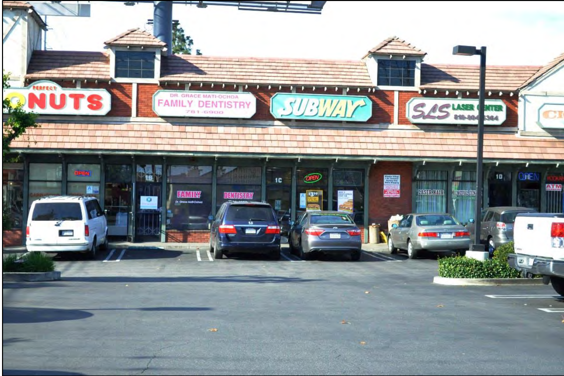
North West Corner of Victory Blvd and Sepulveda Blvd– Commercial Building (Open Air Mall) – DSC0087
