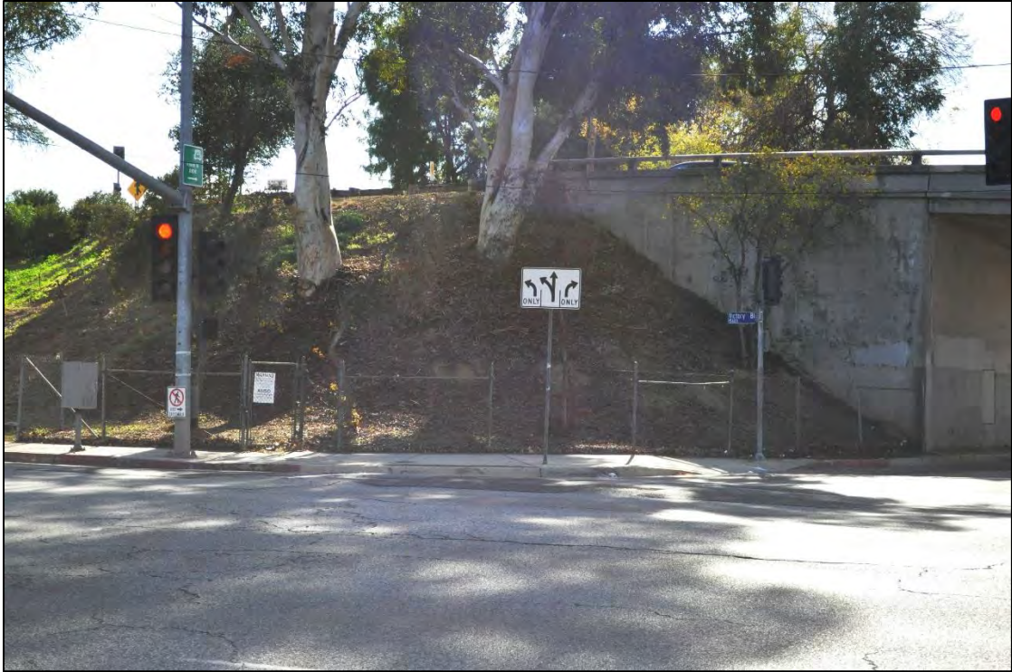
South East Corner of Victory Blvd and Haskell Ave— DSC0095
