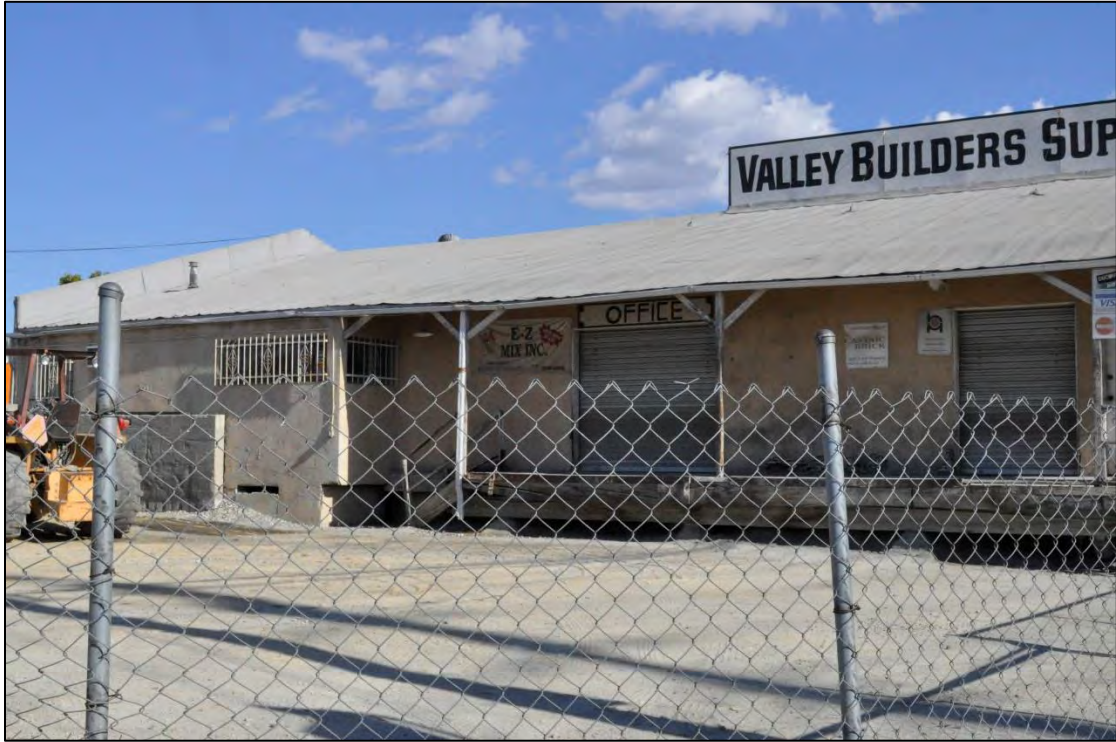
6000 Kester Ave - Commercial building - DSC0109
