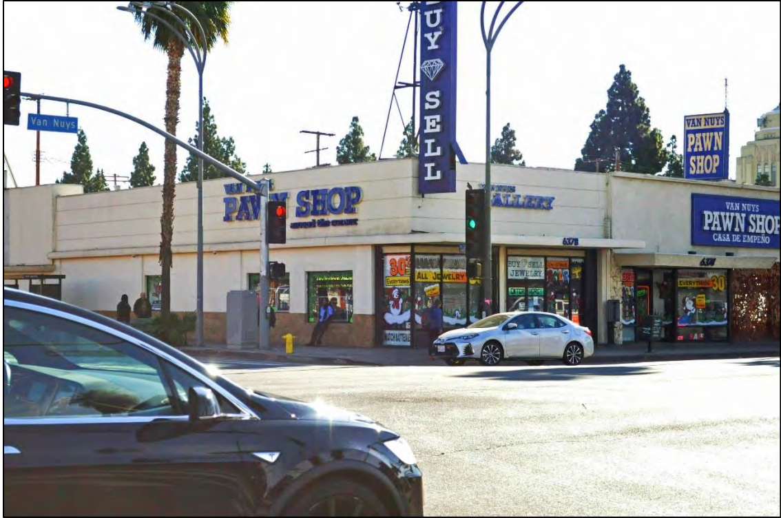
6378 Van Nuys Blvd-South West Corner of Victory Blvd and Van Nuys Blvd – Commercial building - DSC0080
