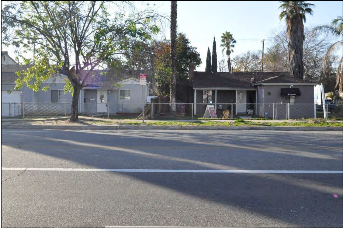
11222 & 11218 Victory Blvd – Single-family homes – DSC0037
