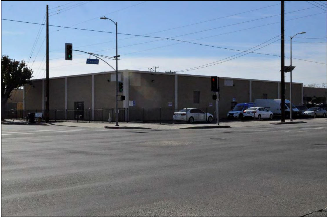
South East Corner of Kester Ave and Oxnard St.- Commercial Building – DSC0111
