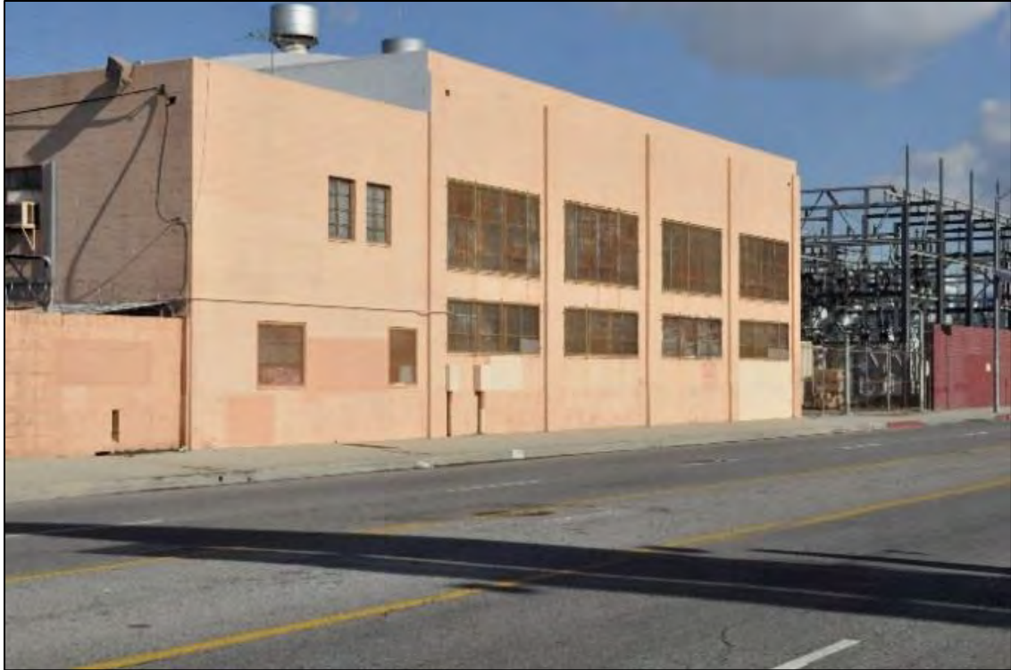
14453 Oxnard St. – Utilities Building - DSC0114
