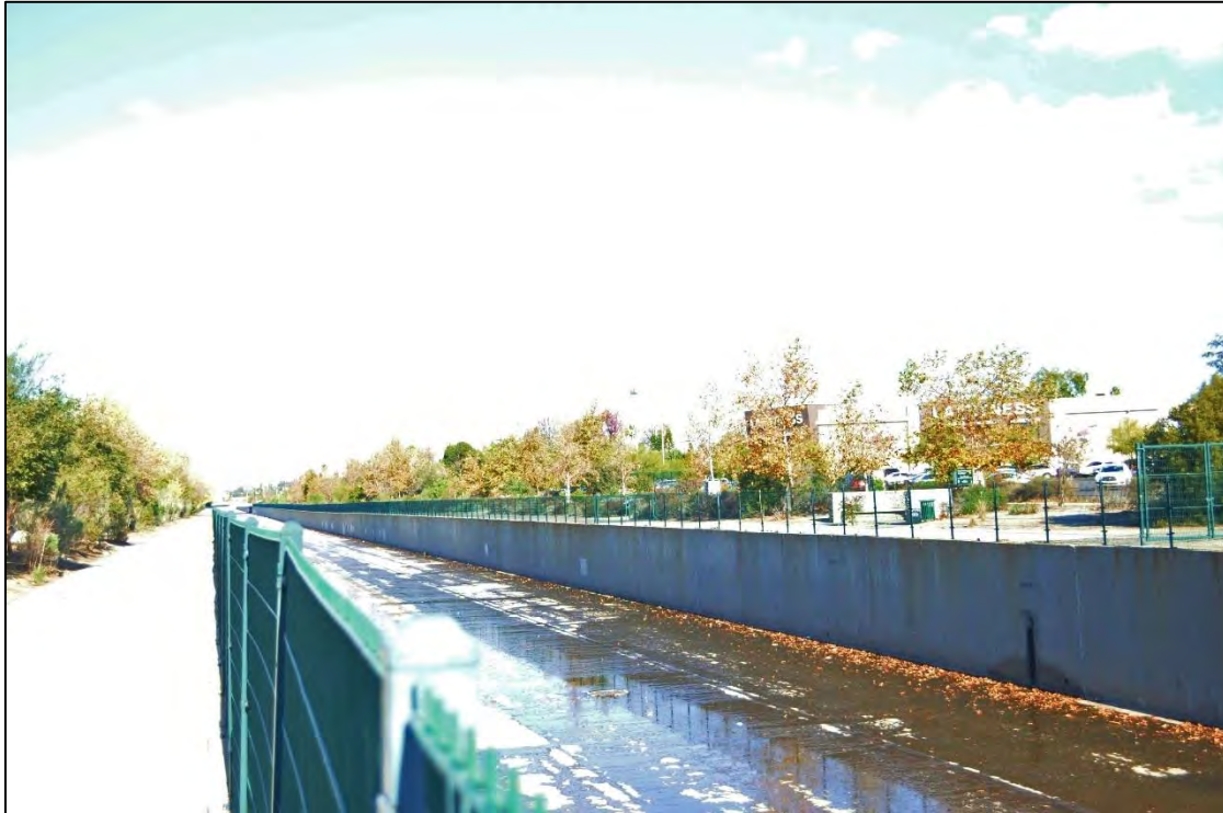
Tujunga Wash Flood Control Channel North of Victory Blvd and west of Coldwater Canyon Ave– DSC0066
