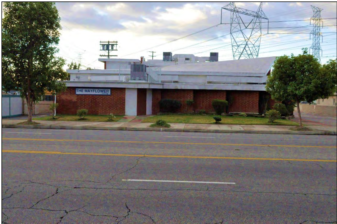
Figure 14. The Mayflower building (11110 Victory Boulevard)
