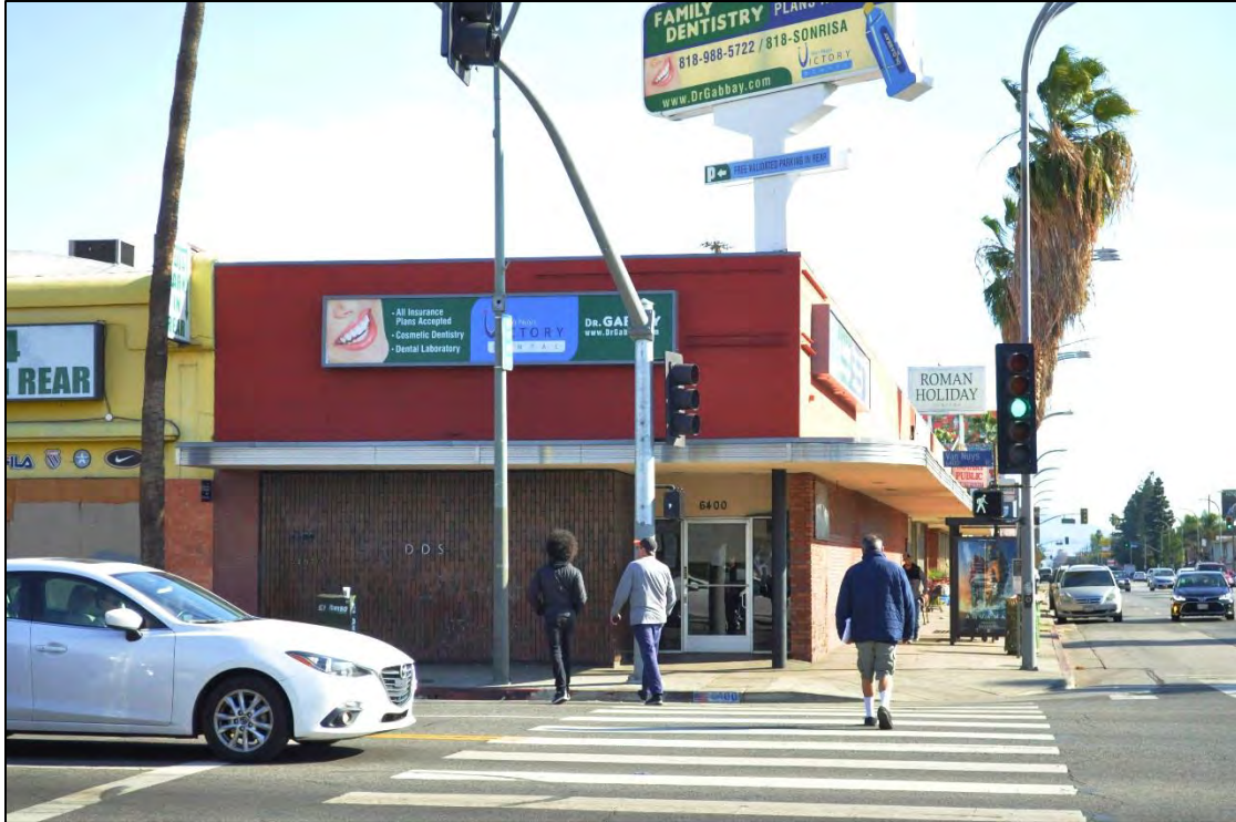
North East Corner of Victory Blvd and Van Nuys Blvd – Commercial Building – DSC0082
