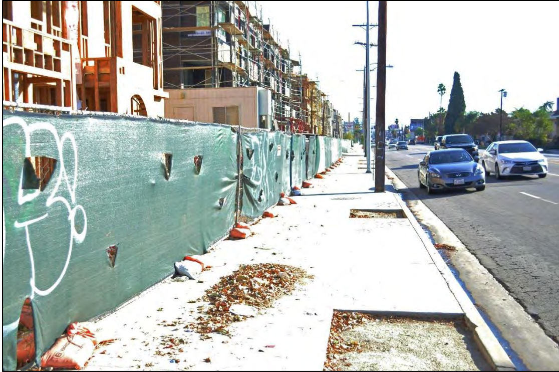
Pump Station Location east of Victory Blvd and Fulton Avenue – DSC0065
