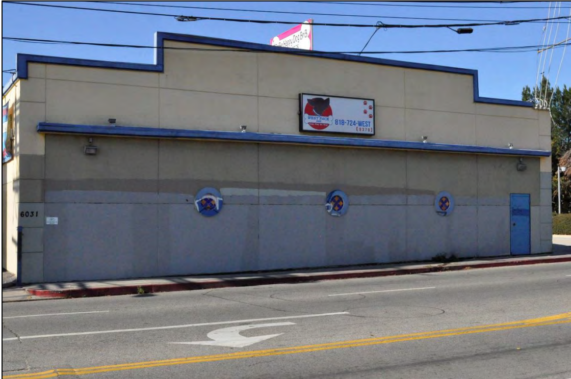
6031 Kester Ave – Commercial Building – DSC0104
