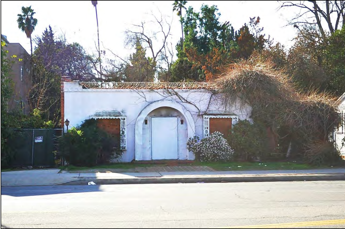
Figure 13. Single family home built in 1923 that resembles a Spanish Colonial Revival architectural type
