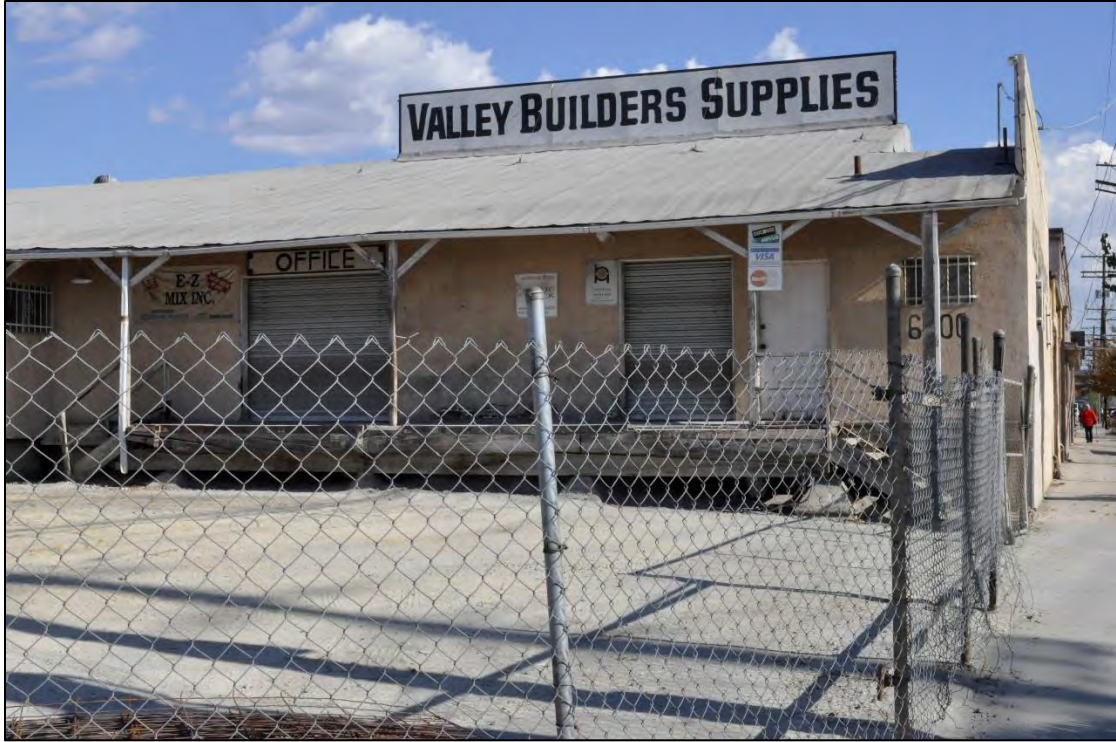
6000 Kester Ave - Commercial building - DSC0109
