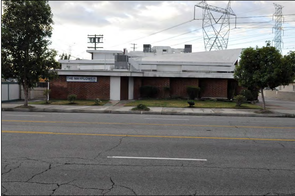
11110 Victory Blvd-The Mayflower – Commercial Building -DSC0024
