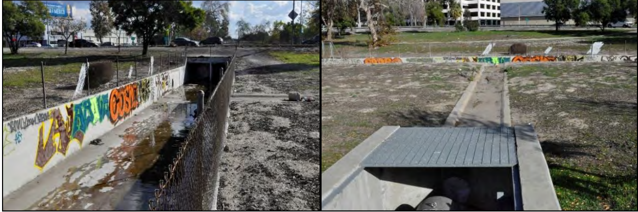
Figure 16. Little Tujunga Wash and Perpendicular culvert located east of State Route 170
