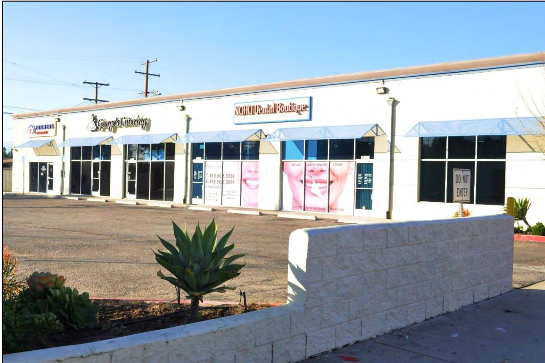
11404 Victory Blvd-South West Corner of Tujunga Ave and Victory Blvd – Commercial Building (Strip Mall) – DSC0045
