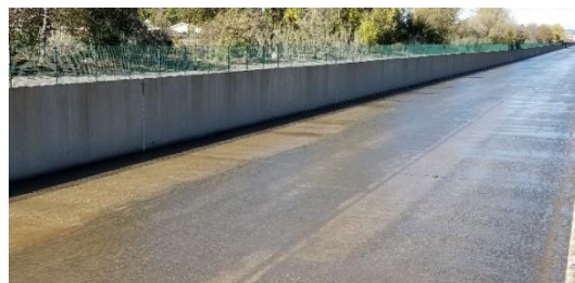
Figure 4. Cement box channel, Tujunga Wash, near Victory Boulevard.
