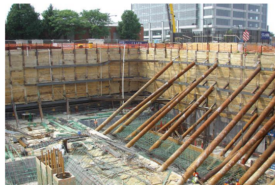
Rakers and tiebacks provide temporary support during construction.
