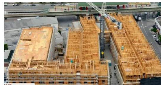
Construction adjacent to the Chinatown Rail Station.
