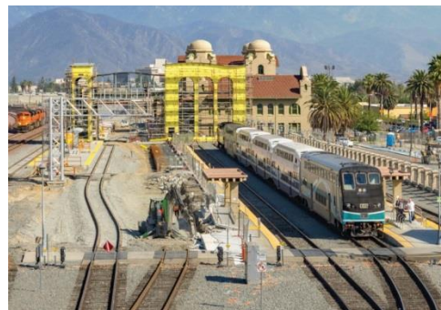
Major construction at the Metrolink San Bernardino Station.
