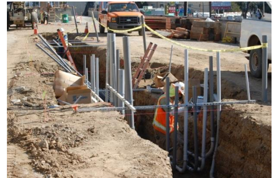
Coordination of underground utilities is critical.
