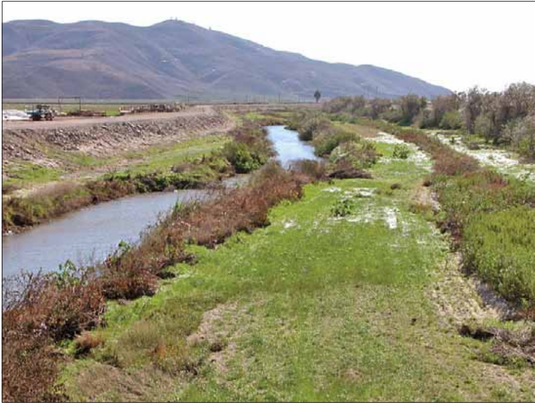
VIEW: Pedestrian/motorist's view of the Oxnard-Camarillo Greenbelt looking south toward Pt. Mugu State Park/Santa Monica Mountains.
