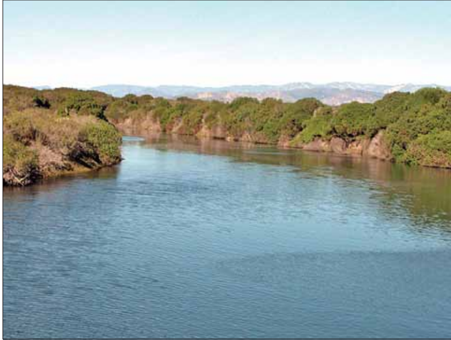
VIEW: Motorist's view of Edison Canal from West Fifth Street.
