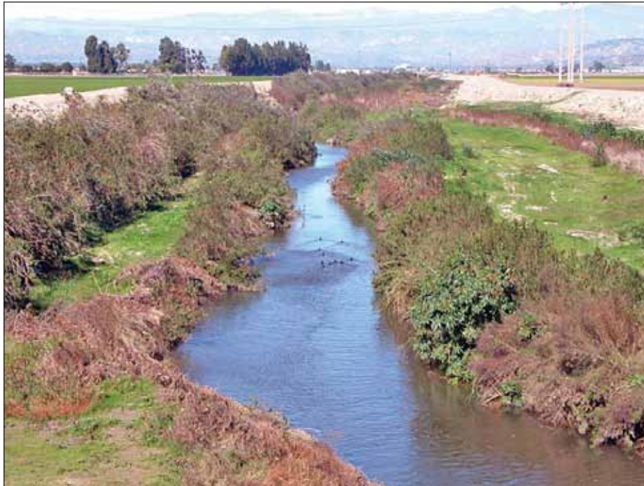
VIEW: Motorist's view of Revolon Channel.
