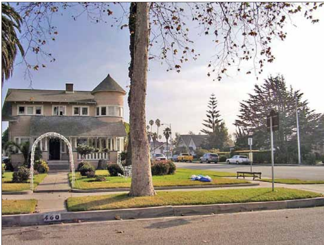
VIEW: Motorist's view of Henry T. Oxnard Historic District.
