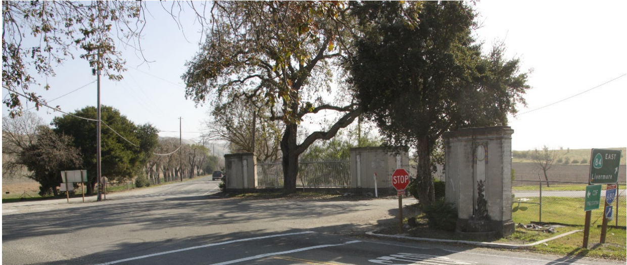
Figure 2.2.9-2. Eastbound SR 84, Paloma Way Tree Allée (Left) and Sunol Water Temple Gates (Right)
