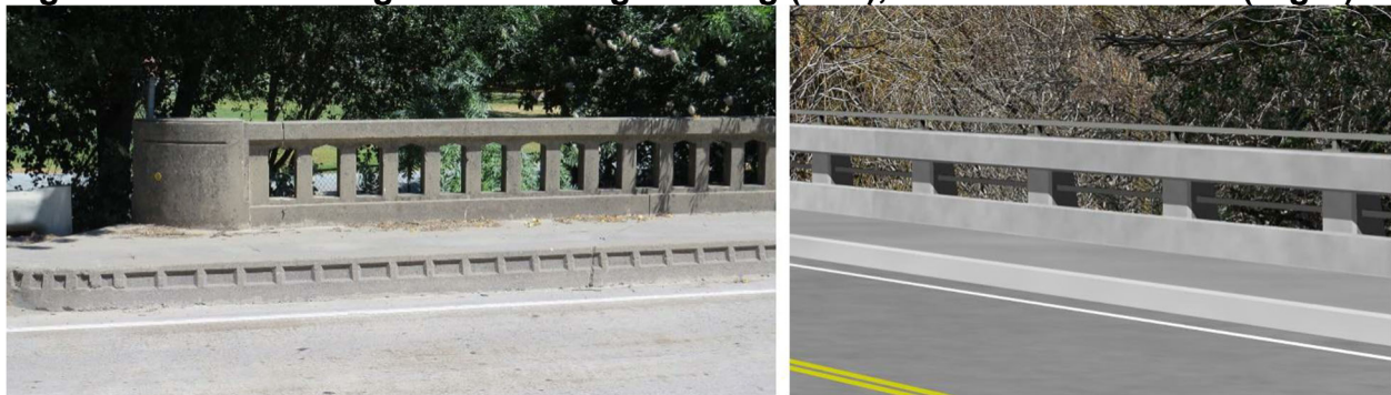
Figure 2.2.9-8. Existing View of Bridge Railing (Left), and Simulated View (Right)
