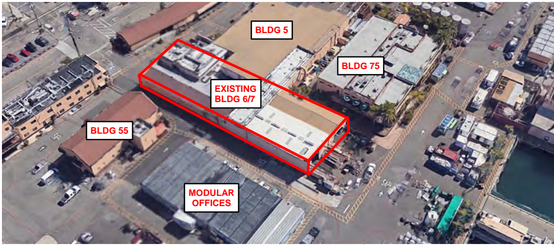
Location of existing bldg 6 & 7 to be demolished in-way-of new production building in similar footprint
