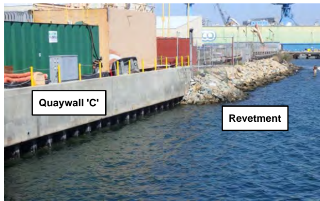
Pier 4 South Quaywall, looking towards south property line
