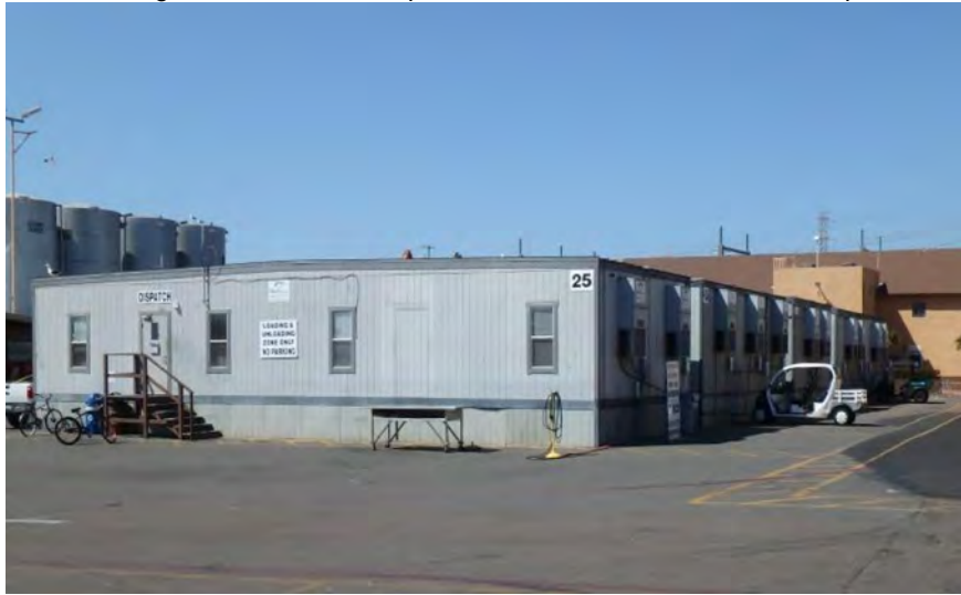
Modular offices to be removed in-way-of administrative office construction
