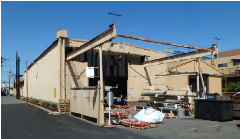
Bldg 6/7 (west) to be demolished in-way-of new prod. bldg.
