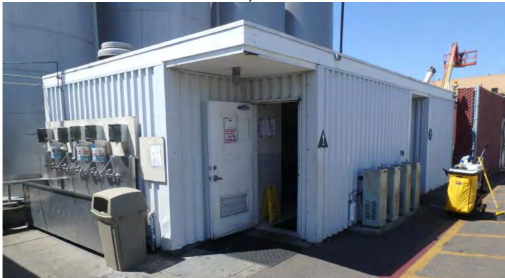
Existing pier 1 restroom to be demolished and incorporated into new admin complex
