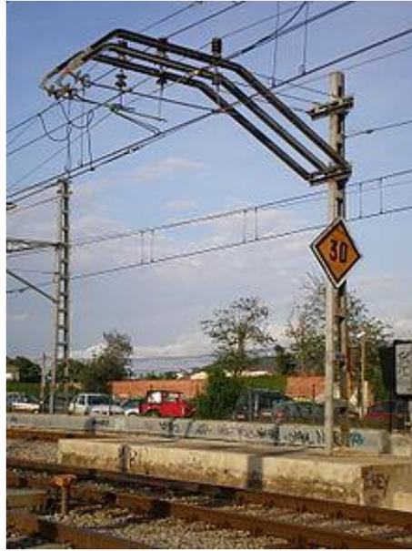
Figure 5. OCS temporary foundation
