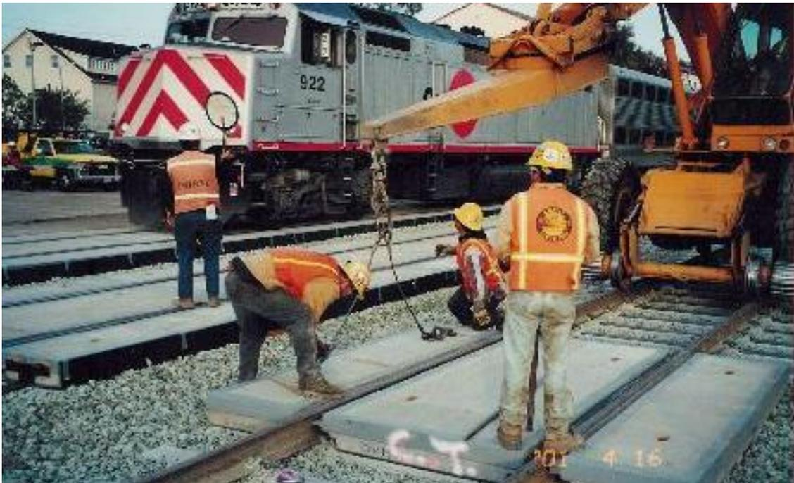
Figure 14. Construction of at-grade crossing
