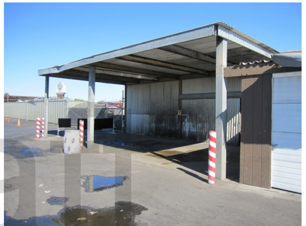
Photograph 12. Steam cleaning area near food services warehouse.
