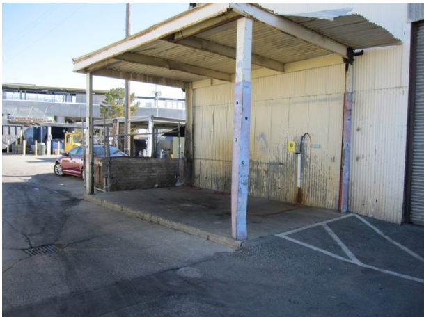
Photograph 13. Steam cleaning area at maintenance building.
