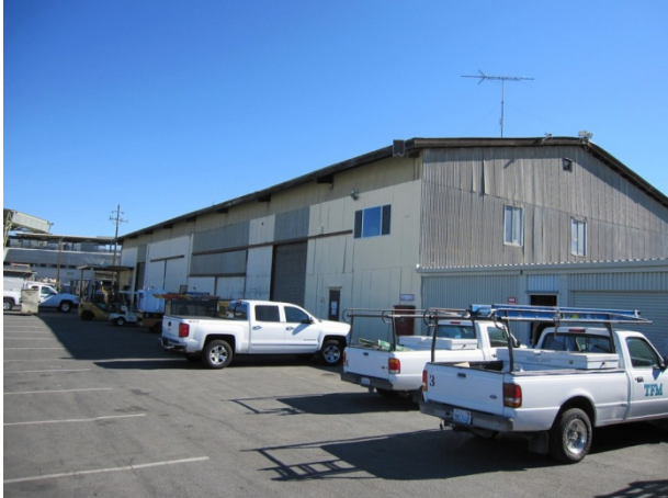
Photograph 3. View of main maintenance building.
