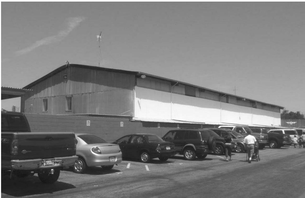
Image 16: slaughterhouse building (southeast corner of site, north of parking)
