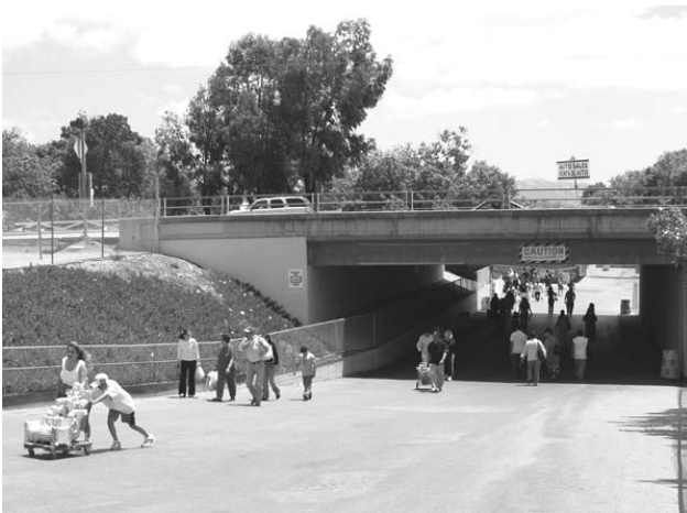
Image 15: underpass viewed from the northwest
