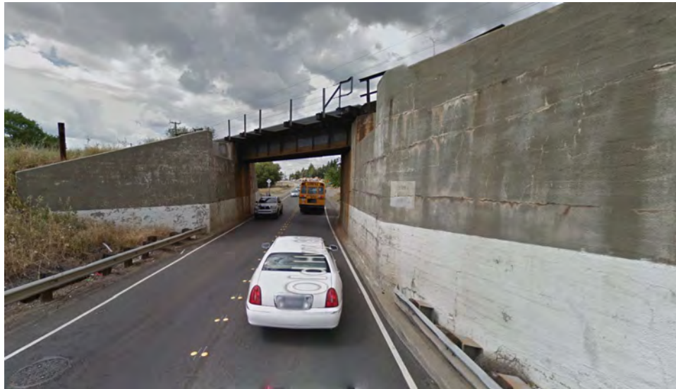
View of northbound Washington Boulevard at UPRR Andora Underpass
