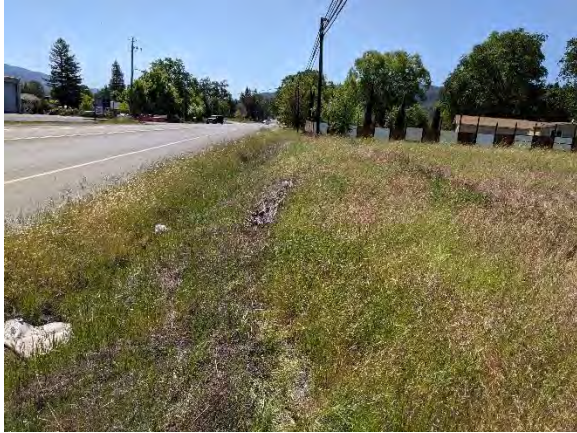
P09 – Upland roadside swale looking south
