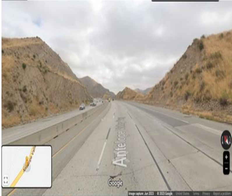
Figure 3. Looking northwest at the steep cut slopes along the SR 14 freeway adjacent to Bee Canyon.
