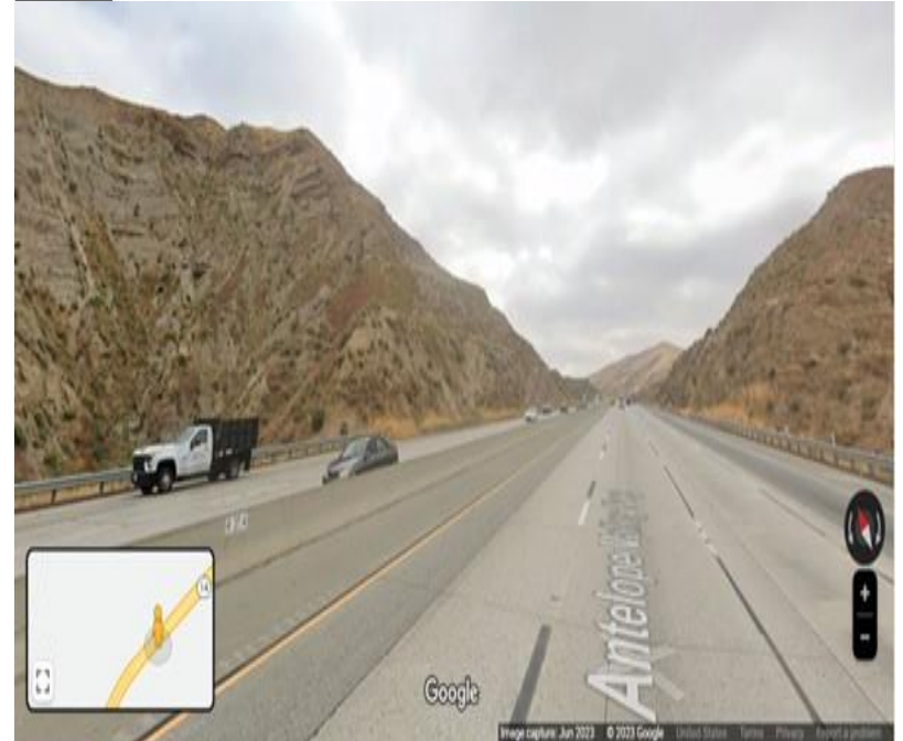
Figure 4. Looking northwest at the steep natural terrain and steep road cuts along the SR 14 freeway adjacent to Bee Canyon.
