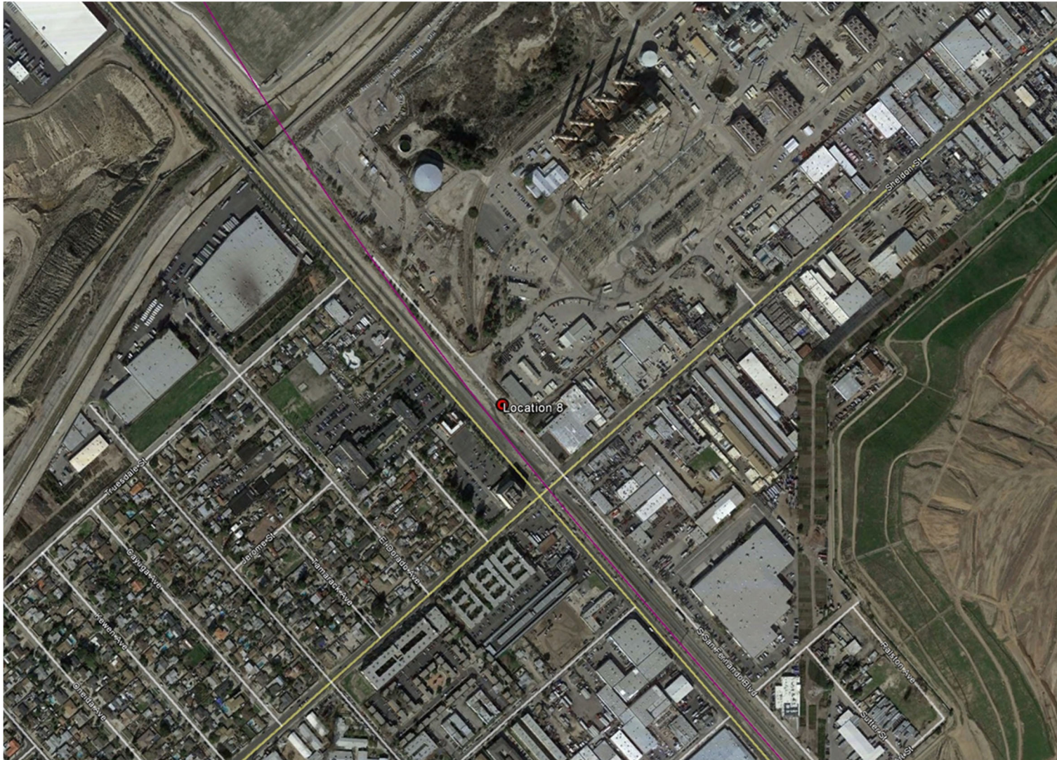
Figure B3.5-8(a) Location 8: San Fernando Boulevard, Sun Valley Urban setting adjacent to medical center and near the existing rail alignment (Lat 34.241189°, Lon -118.394963°)
