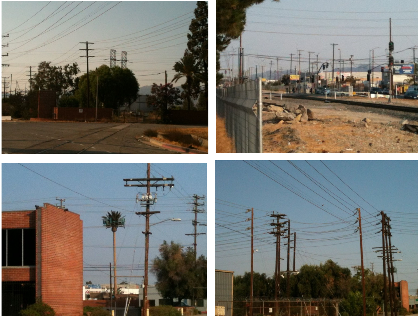
Figure B3.5-8(c) Location 8: San Fernando Boulevard, near Sheldon Street, Sun Valley Nearby emitters include HV transmission lines, distribution lines, and cell towers
