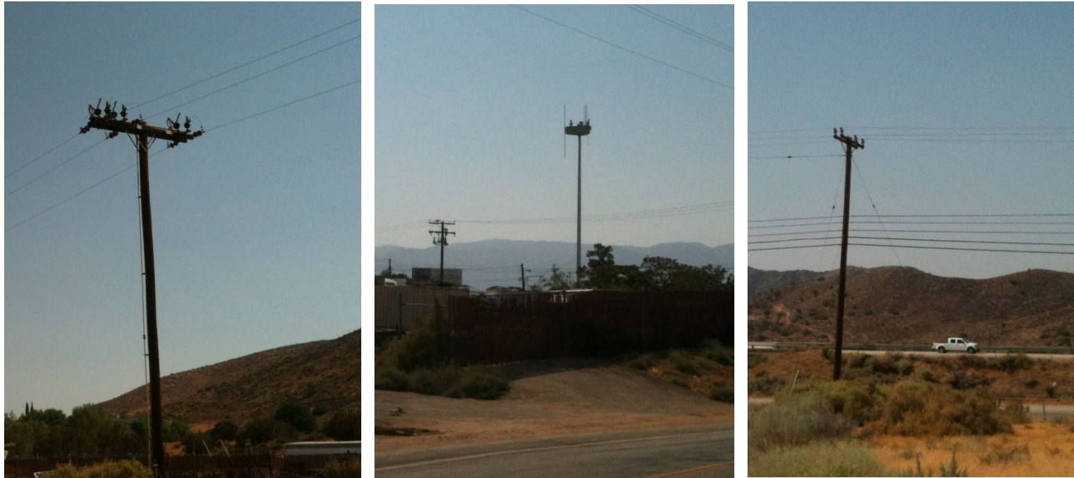
Figure B3.5-5(c) Location 5: Red Rover Mine Road, near Sierra Highway, Acton
