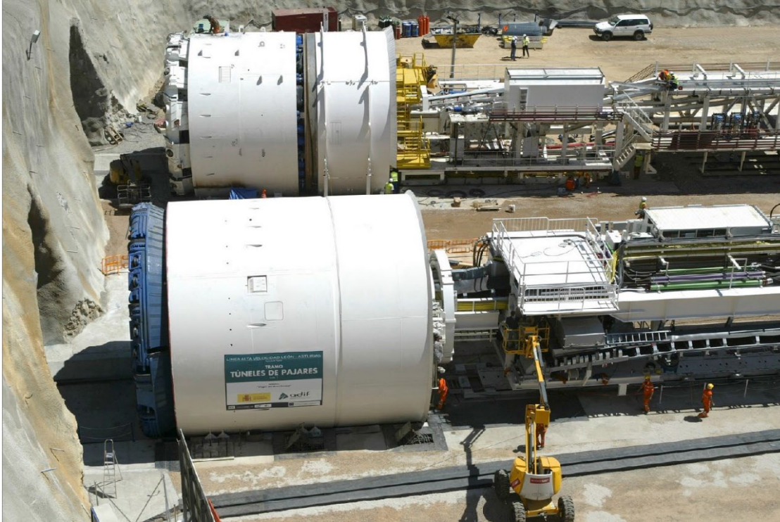
Figure 2-104 Tunnel Boring Machines at a Double Portal Entrance
