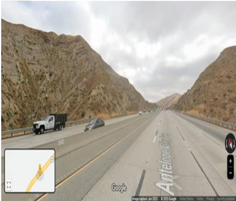
Figure 5. Looking northwest at the steep natural terrain and steep road cuts along the SR 14 freeway adjacent to Bee Canyon.
