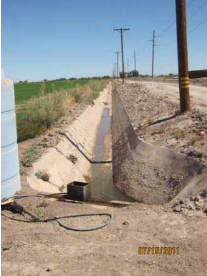
IMG_1851 Wormwood Lateral 7 at West Diehl
