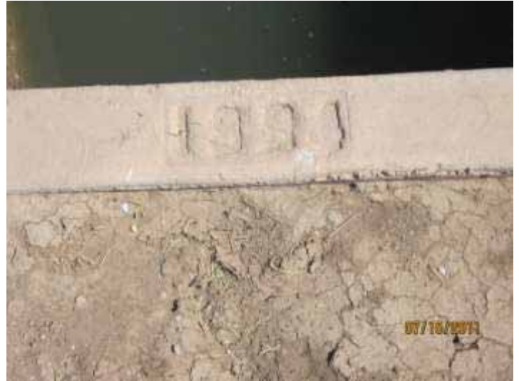
IMG_1850 Wormwood Canal at West Diehl
