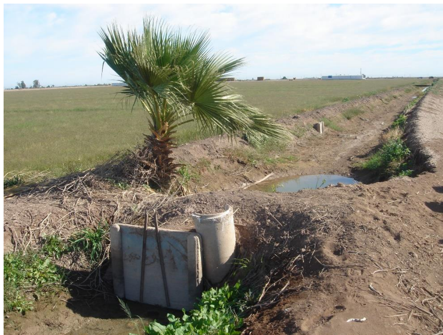
Figure 5. DS-I-2 – Overview of canal and concrete gate looking northeast, 11/20/17, IMG_00008.
