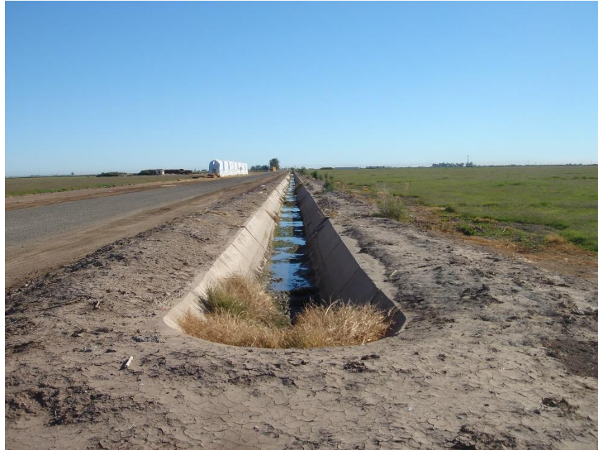
Figure 8. P-13-013073 – Overview of concrete lined canal looking east, 11/21/17, IMG_00046.
