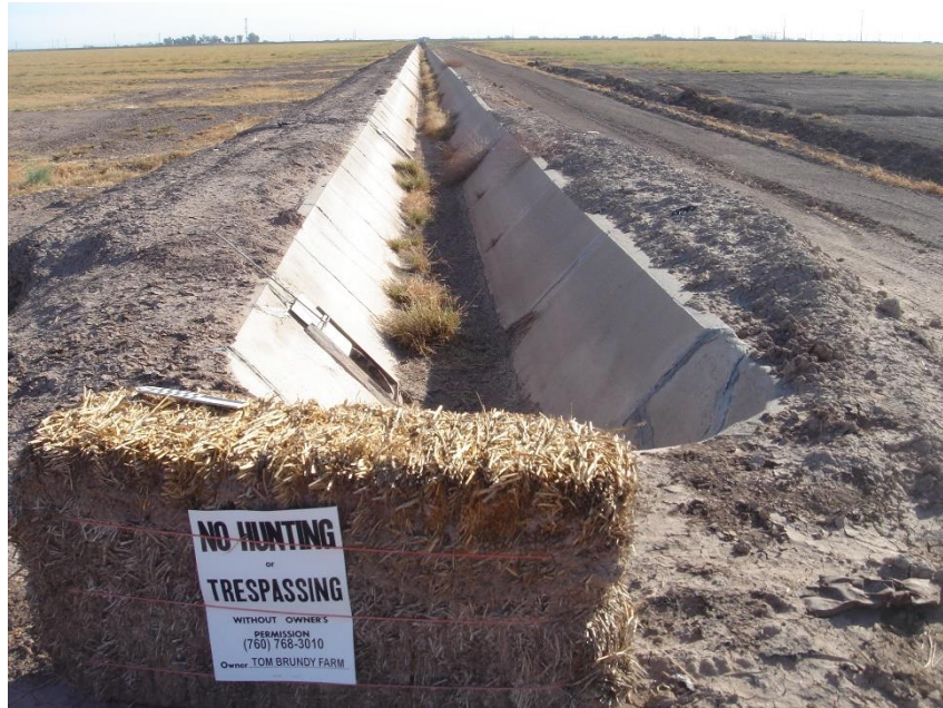
Figure 7. DS-I-4 – Overview of canal looking east, 11/20/17, IMG_00028.
