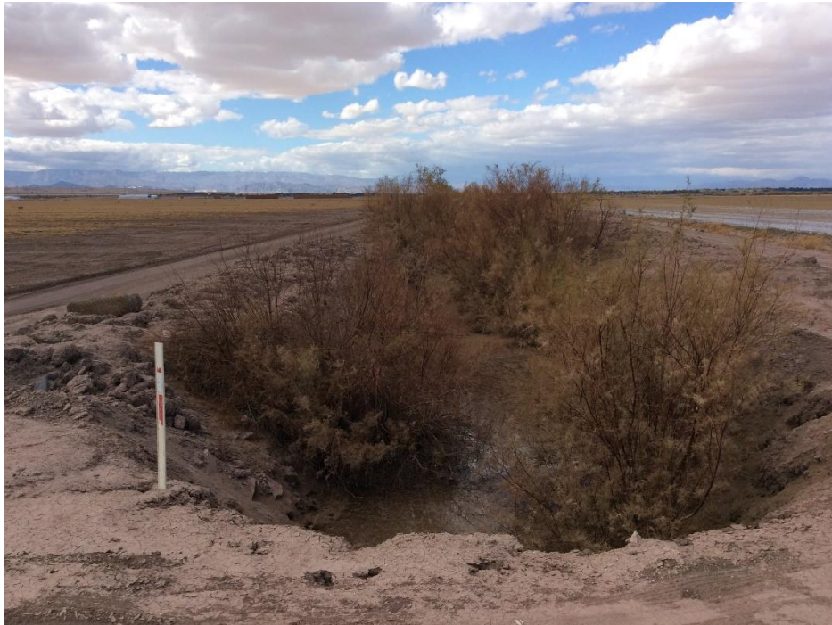
Figure 11. DS-I-8– Overview of drain looking east, 2/22/18 (IMG_0341)).
