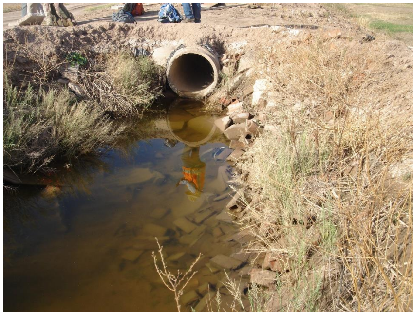
Figure 4. DS-I-1 – Overview of canal and concrete pipe drain looking west, 11/20/17, IMG_00001.
