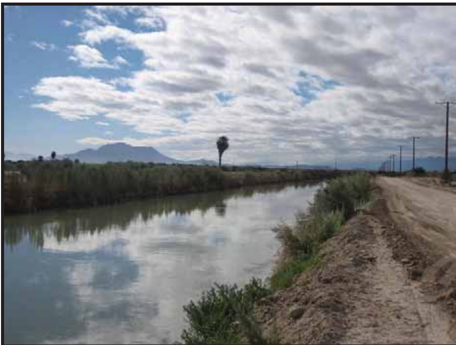
Westside Main Canal, View to the South
