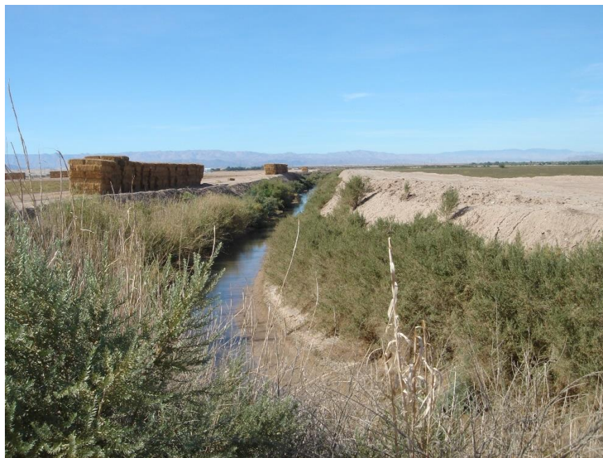
Figure 9. P-13-013079 – Overview of drain looking west, 11/21/17, IMG_00042.
