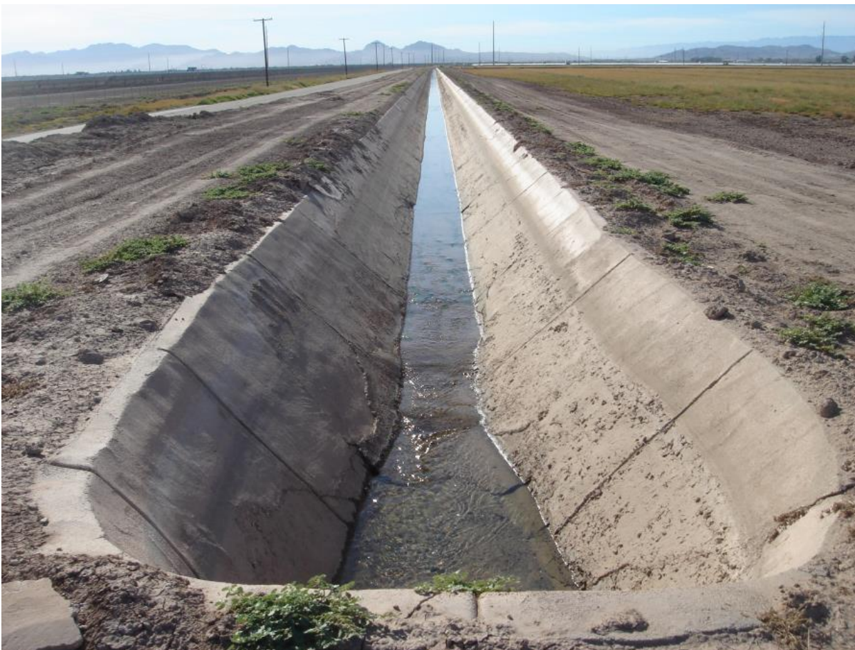
Figure 10. P-13-013074 – Overview of canal looking south, 11/21/17, IMG_00036.
