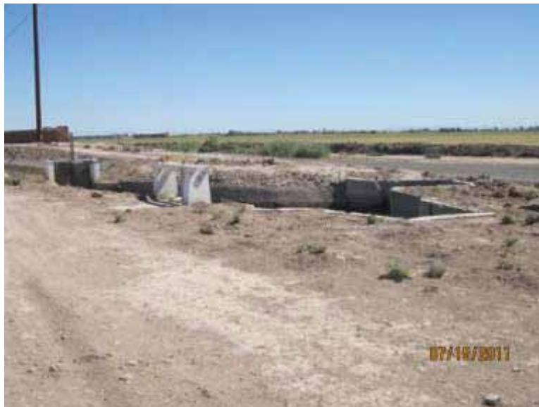
IMG_1849- View to NNE Wormwood Canal at West Diehl Road.
