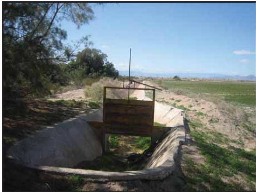
At the origin of the east-west portion of WSM Pump 6, looking west at the metal check
