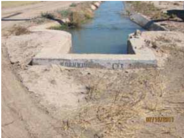
IMG_1846-view to north Wormwood Lateral 7 at Wixom Road
