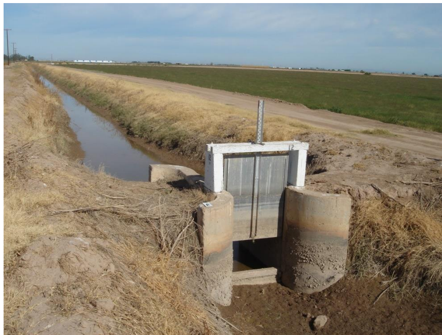
Figure 6. DS-I-3 – Overview of canal and gate 12 looking northeast, 11/20/17, IMG_00017.
