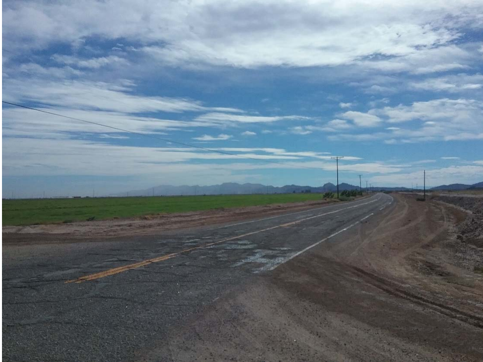
Photo 1: Looking south from the corner of Kubler and Drew Road intersection.
