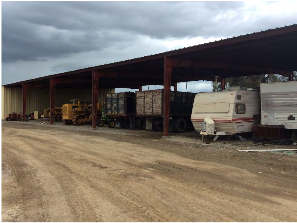
Photograph 1: View of the project site from the east; facing northwest.
