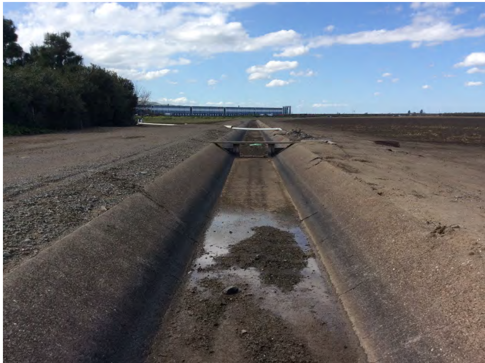
Photograph 6: View of southern portion of aqueduct in APN 021-023-031; facing north.
