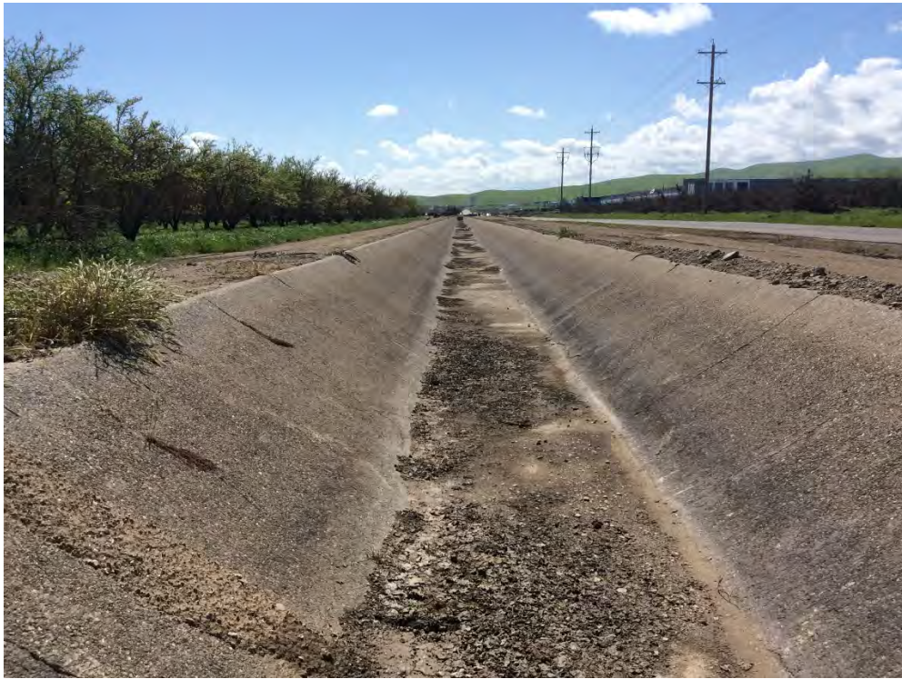
Photograph 7: View of the canal from the north; facing south.
