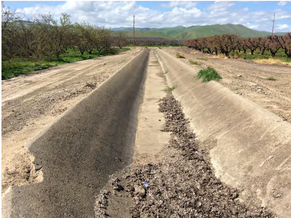
Photograph 6: View of canal facing west
