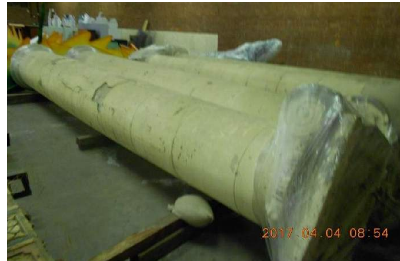
Figure 11. Terra cotta columns. Source: Jergins Trust Artifact Inventory, 4/4/17, courtesy of GBD Architects.
