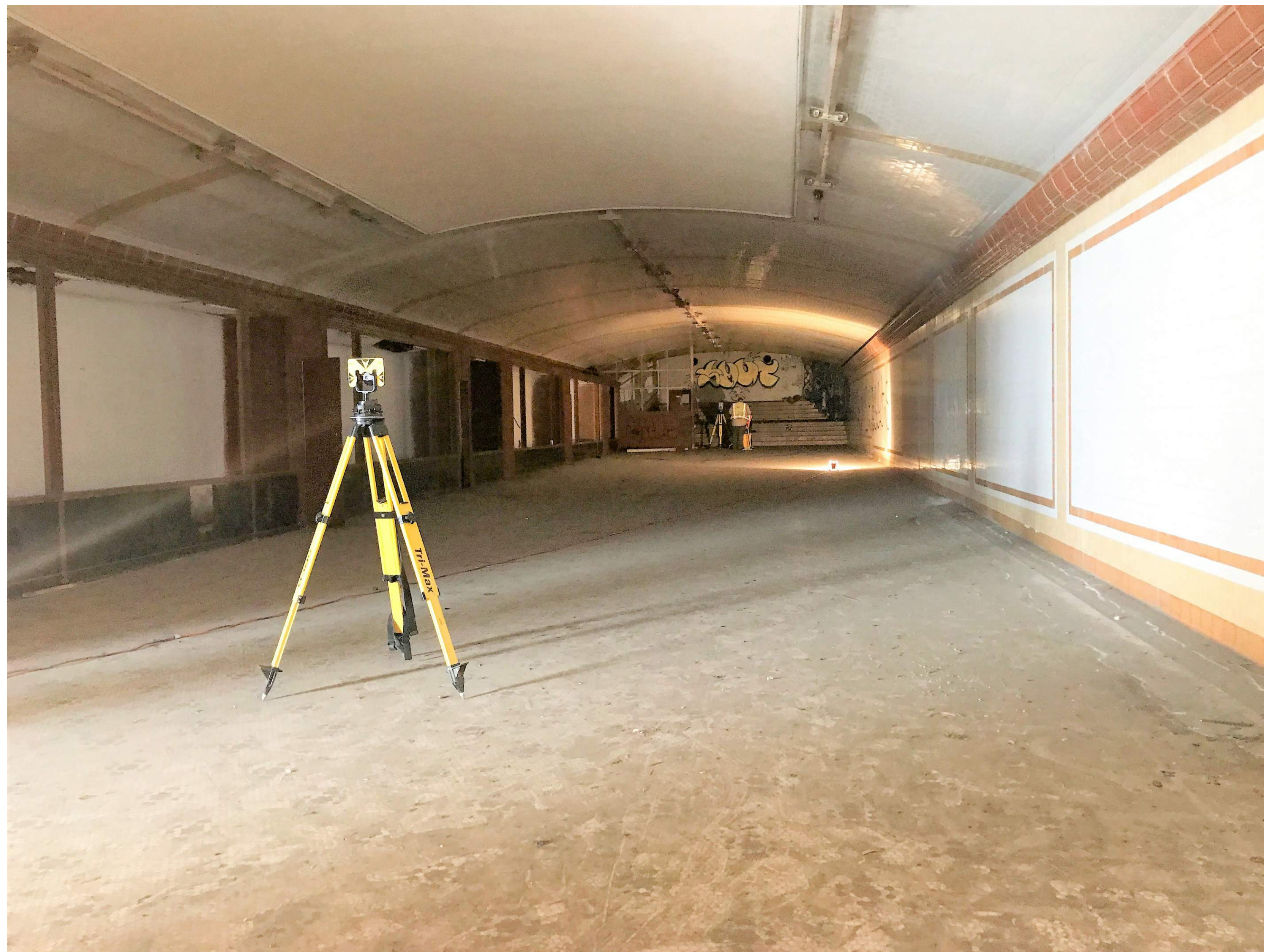
Figure 1. Jergins Tunnel, looking north, May 2018. Source: Page & Turnbull
