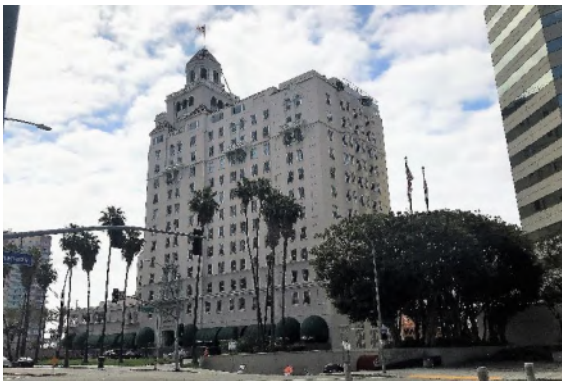
Figure 6: The Breakers at Ocean Boulevard, looking southeast.
