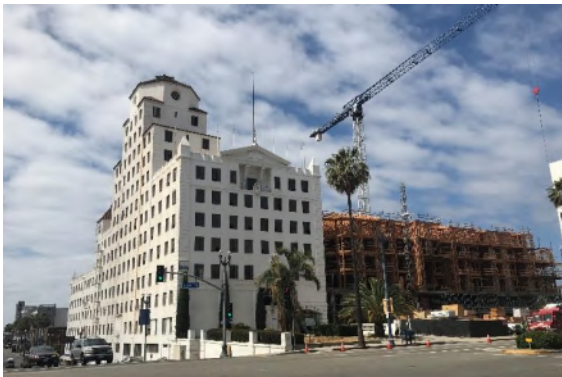
Figure 4: Ocean Center Building at Ocean Boulevard, looking south. Note the Oceanaire development under construction to the west.
