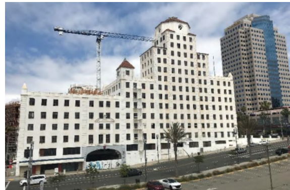
Figure 5: Ocean Center Building along Pine Avenue, looking west. Note the building's different stepped heights and the response to the sloped site.
