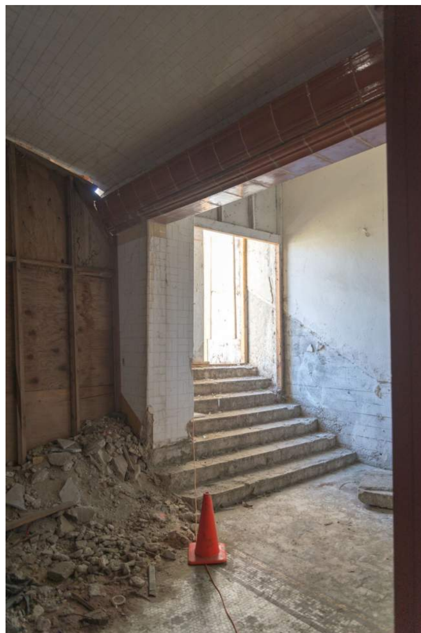
Figure 19. SW entry stair to tunnel, 2016. Source: Michael Wada / Grunion Gazette.
