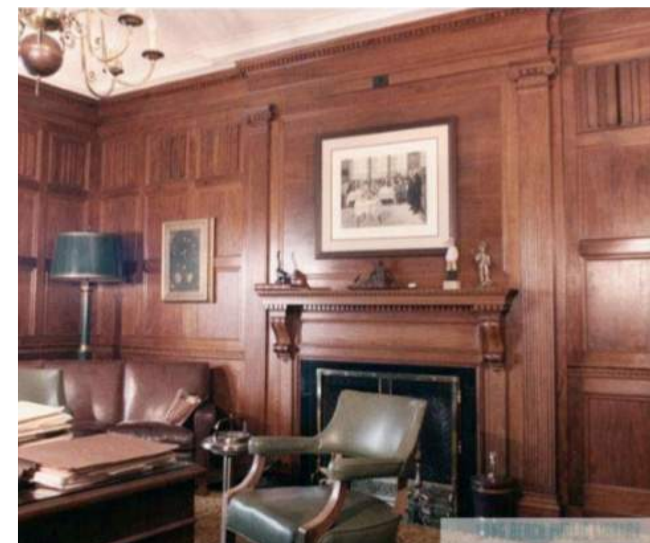
Re-create a single wall based on available historic photographs and artifacts, such as the wall with the fireplace mantel, corbels and pilaster. Source: ESA Report, 2017.
