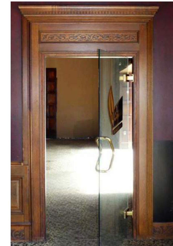
Figure 15. Door frame millwork. Source: ESA Report, 2017.
