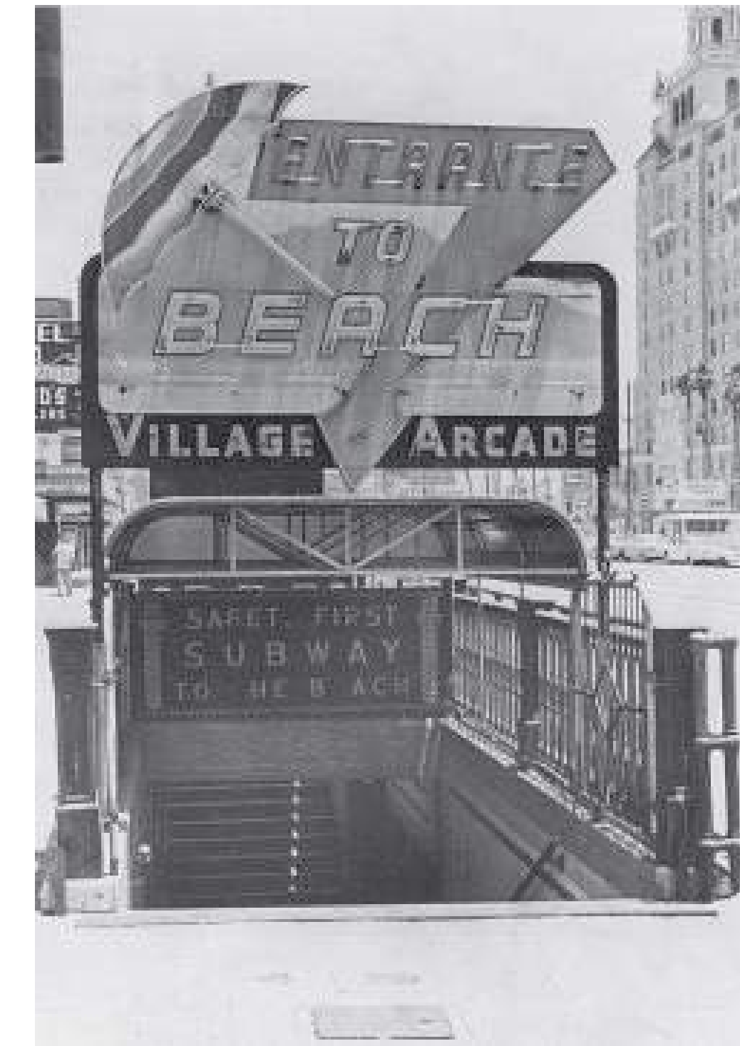
Street entrance to Jergins Tunnel. Source: www.gazettes.com.
