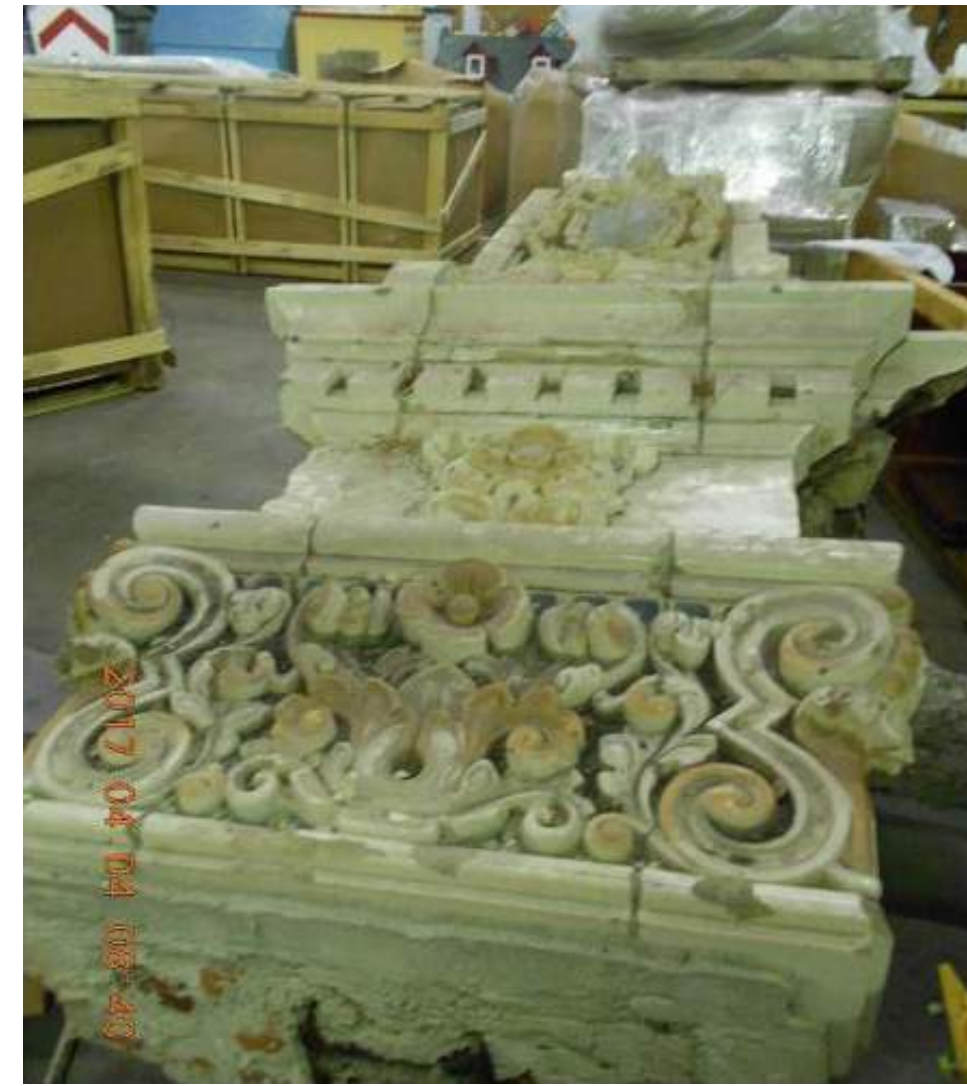
Figure 12. Typical terra cotta piece from parapet. Source: Jergins Trust Artifact Inventory, 4/4/17, courtesy of GBD Architects.
