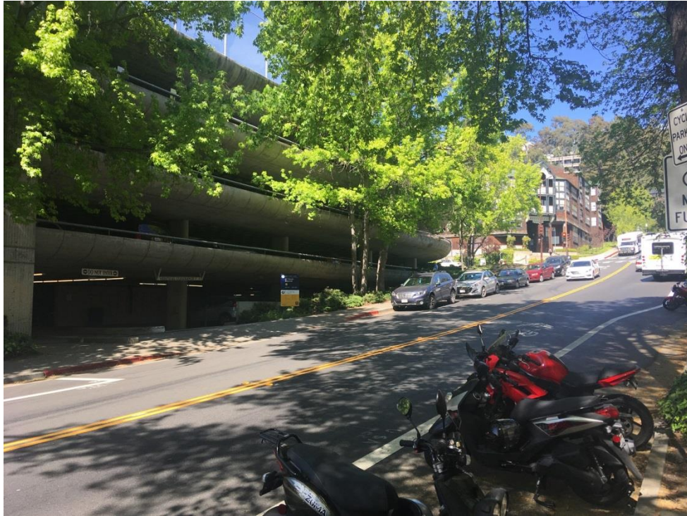
View of Upper Hearst parking structure looking northeast from Hearst Avenue.
