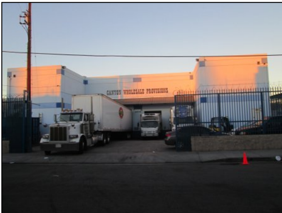
Western Adjoining Property (2)
