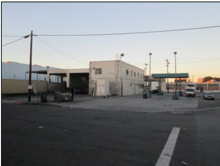
Western Adjoining Property
