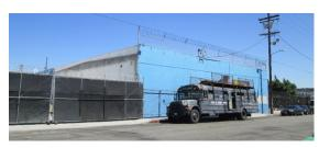
The parcel at 528 S. Seaton Street is occupied by an industrial building developed in 1985. The building is situated along the west, south, and east property lines. The building is rectangular in plan and one story in height. It has a flat roof covered in rolled asphalt. The exterior is brick. There is one garage opening with a roll down metal door offset
